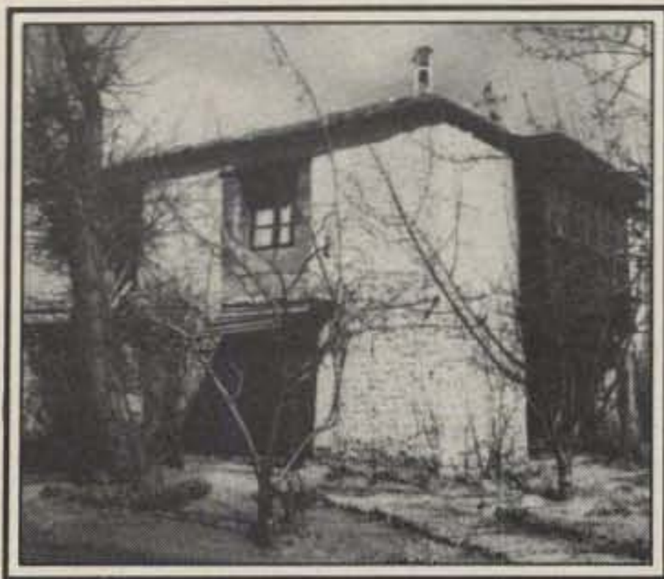
The Consulate General of India where Shankar installed the radio station. He and Namita lived here. The altitude of this spot is 15,000 feet.
