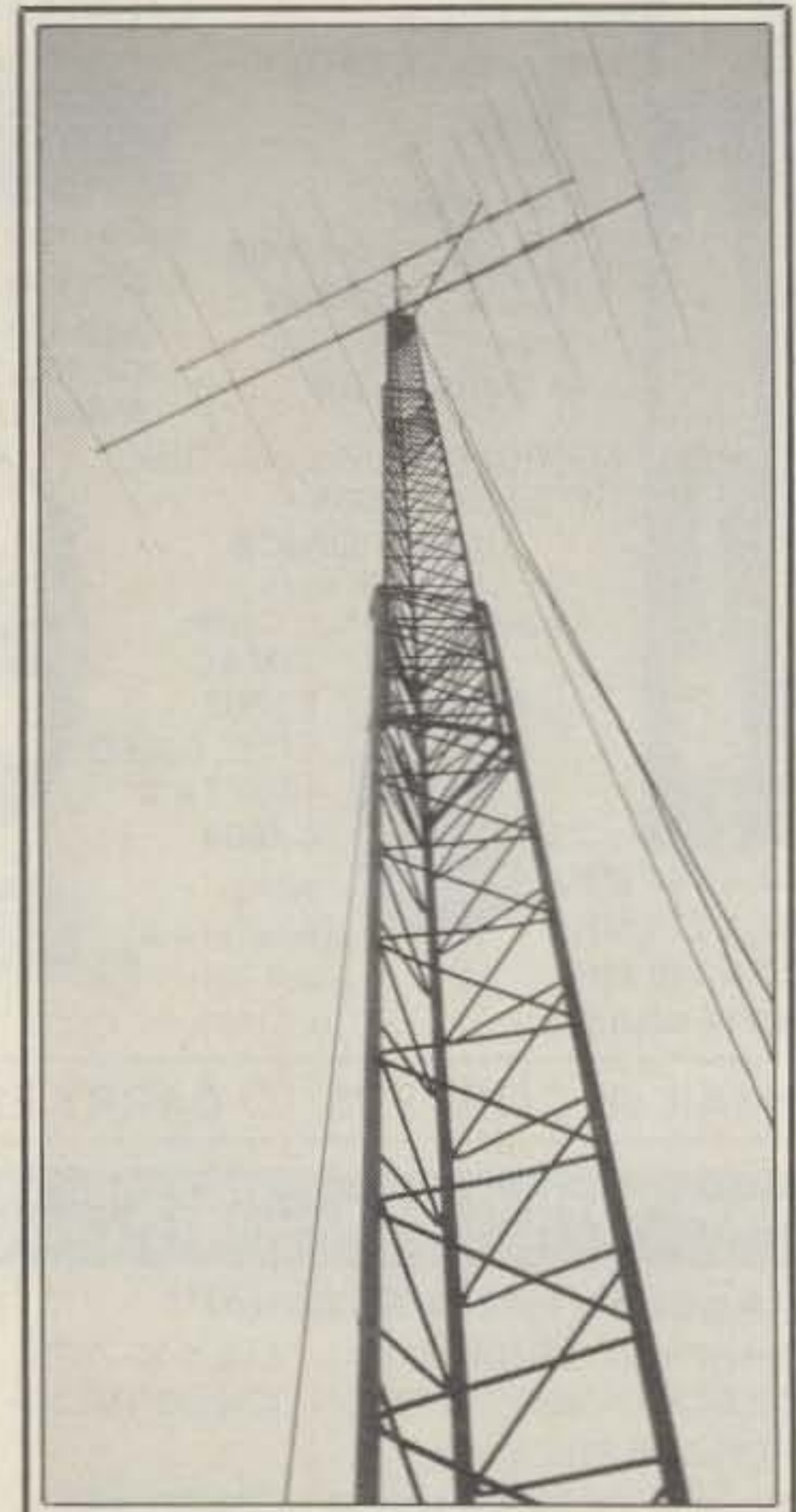
The main 50 MHz antenna system at NV6O/2: a pair of 7 element KLM Yagis at 54 and 70 feet. Second 6 meter antenna was a single 7-element KLM at 50 feet, on a separate tower.
