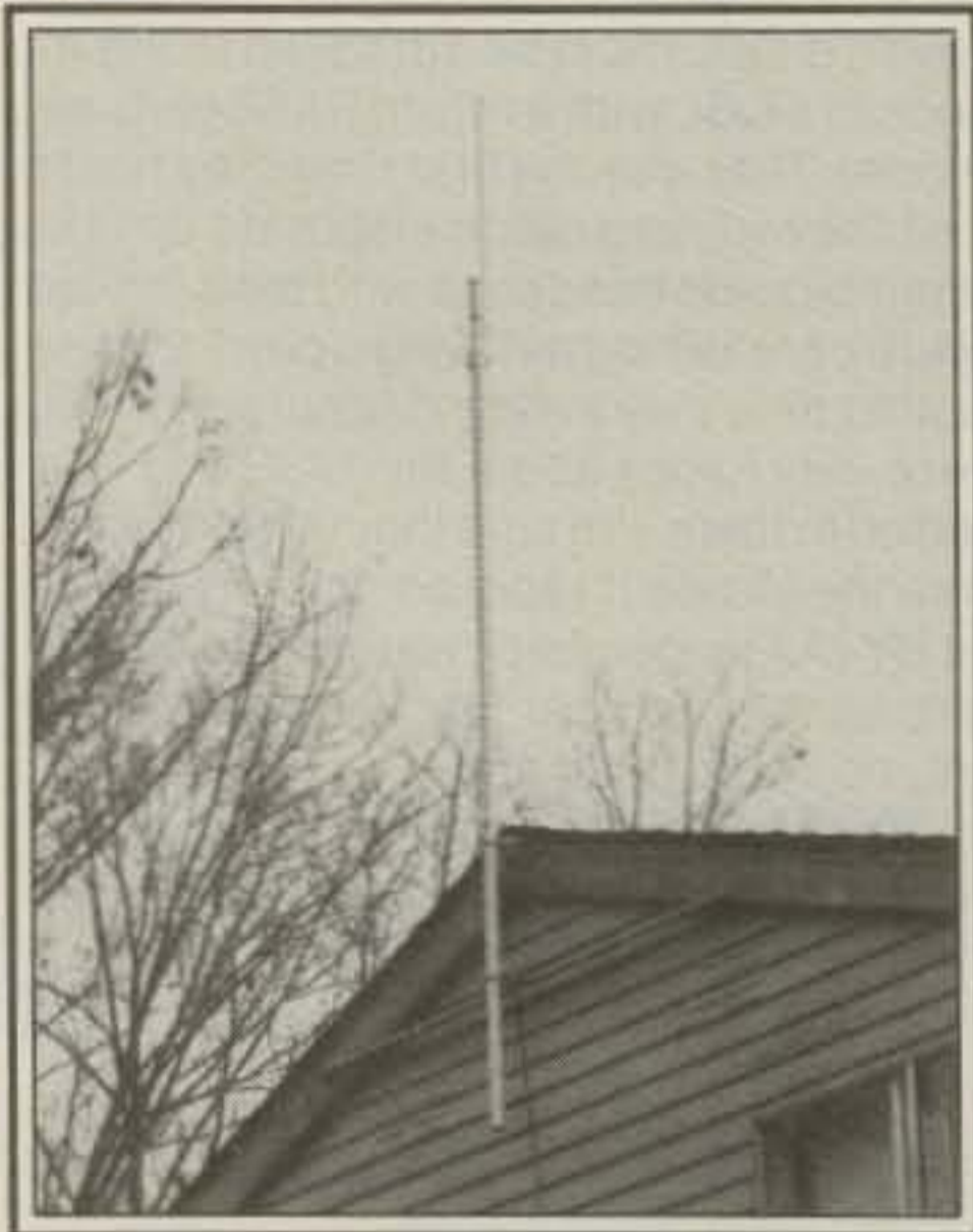
The completed 20 and 30 meter vertical antenna mounted on the author's roof.
