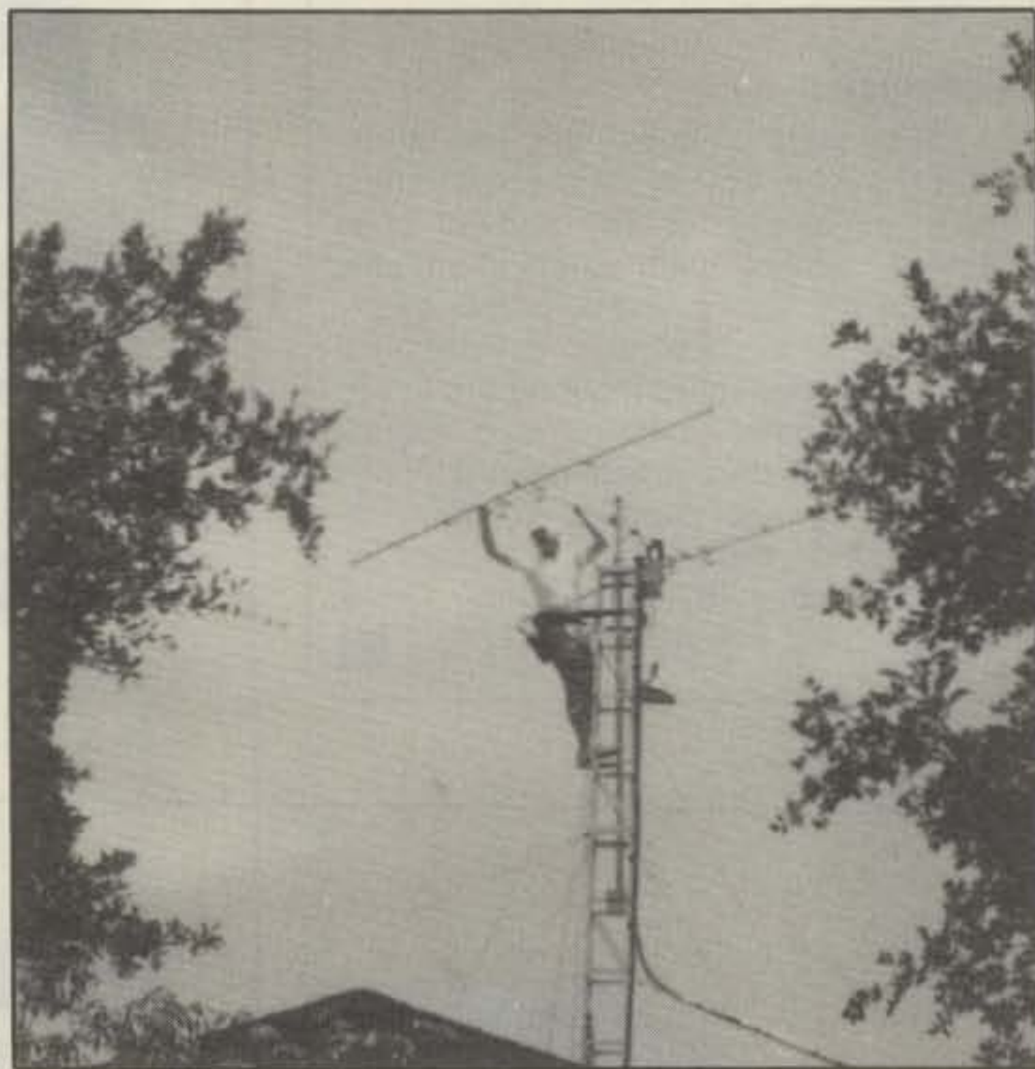
Here is the HF4B ready to be installed. The antenna is so light that it is very easy to manage and work on.
