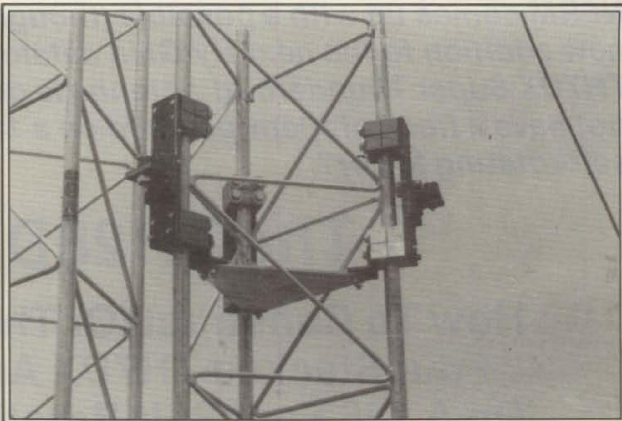
Fig. 3—The tower-mounted fittings for the cam followers. The under and sideways followers are shown installed. The mounting hole for the downward follower can be seen.
