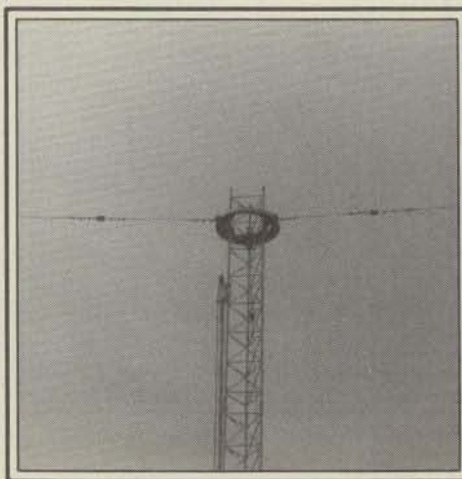
Fig. 12— The first bearing ring is shown in place with its guy wires attached.
