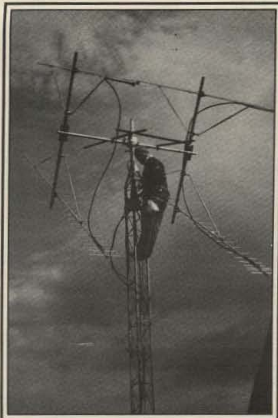
Lanny Aldrich, K1LEC, makes a final adjustment on the NC11/1 70 cm EME array.
