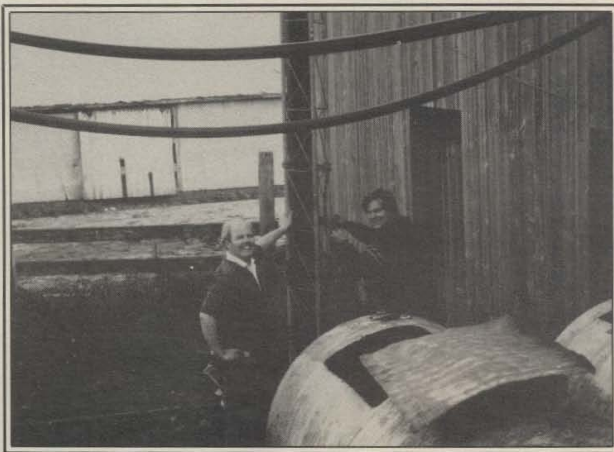
Lanny, K1LEC, and Frank, NC11, lashing a section of Rohn #25 tower to the steel I-beam used for support during the NC11/1 EME expedition to VT.
