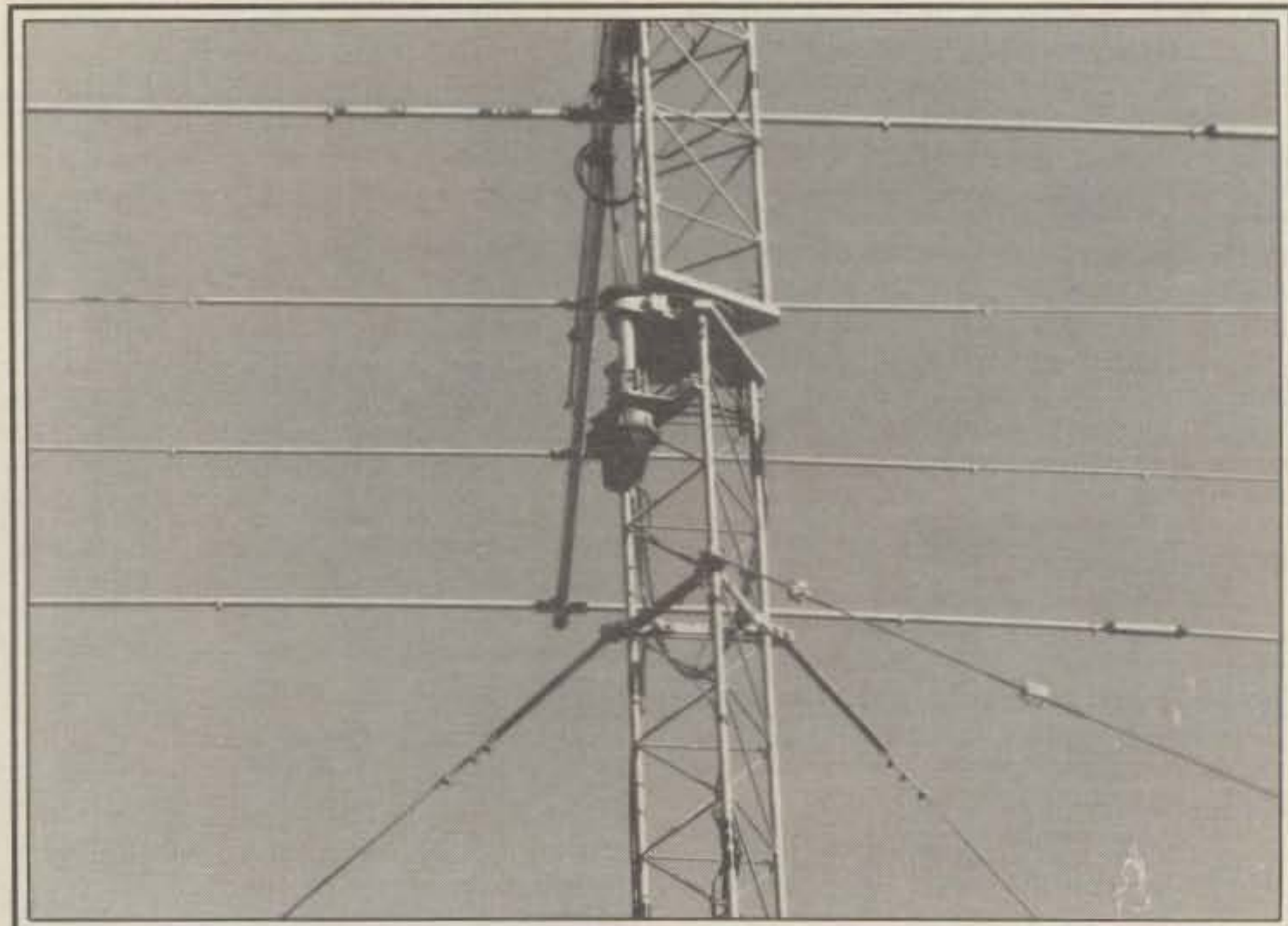
Photo shows the "guts" of the K5IU Rotating Tower System. The rotor can be seen in the foreground. A 2:1 chain drive with the HDR-300 rotor yields 10,000 inch-pounds "turning torque."
