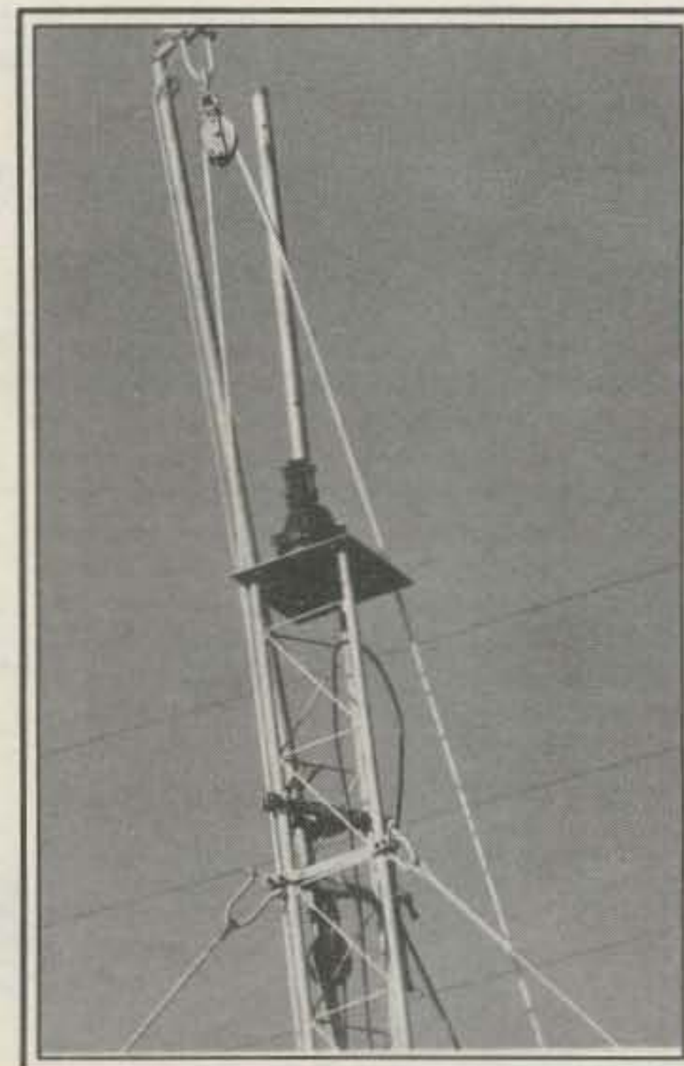
This view shows a bit more clearly how the base plate fits on the top of the tower. Note also that a temporary pulley arrangement has been put in place to lift the antenna.
