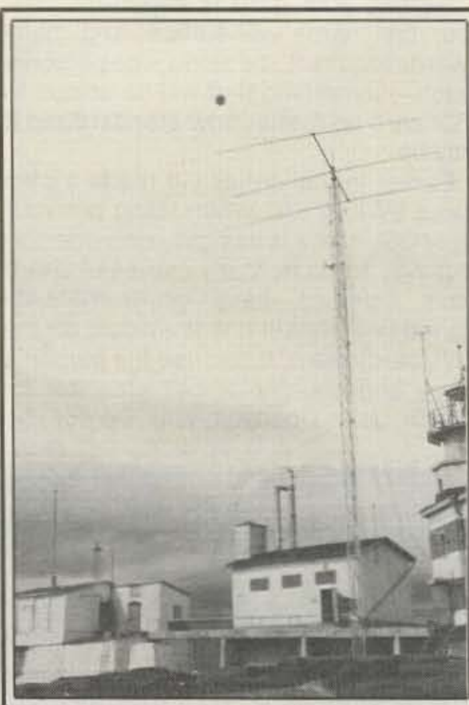
Running beams this close to each other and operating two kw rigs on the same band was proof of technical excellence. Don't get it wrong—it wasn't this calm very often. The balloon in the background supported the 160 meter vertical.
