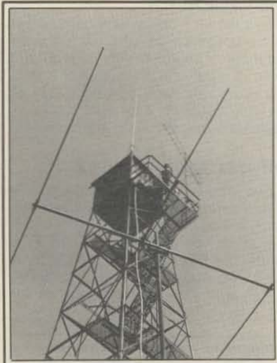
Who's that up there? This is the site of WW4T/3, FNO1, the only WW3 prefix in the July VHF WPX Contest. The gang did a bang-up job, operating from this 85 foot fire tower atop a 2400 foot mountain in western PA. The 144 and 432 MHz antennas are above the tower; the 3-element 6 meter beam was on its own 20 foot mast.
