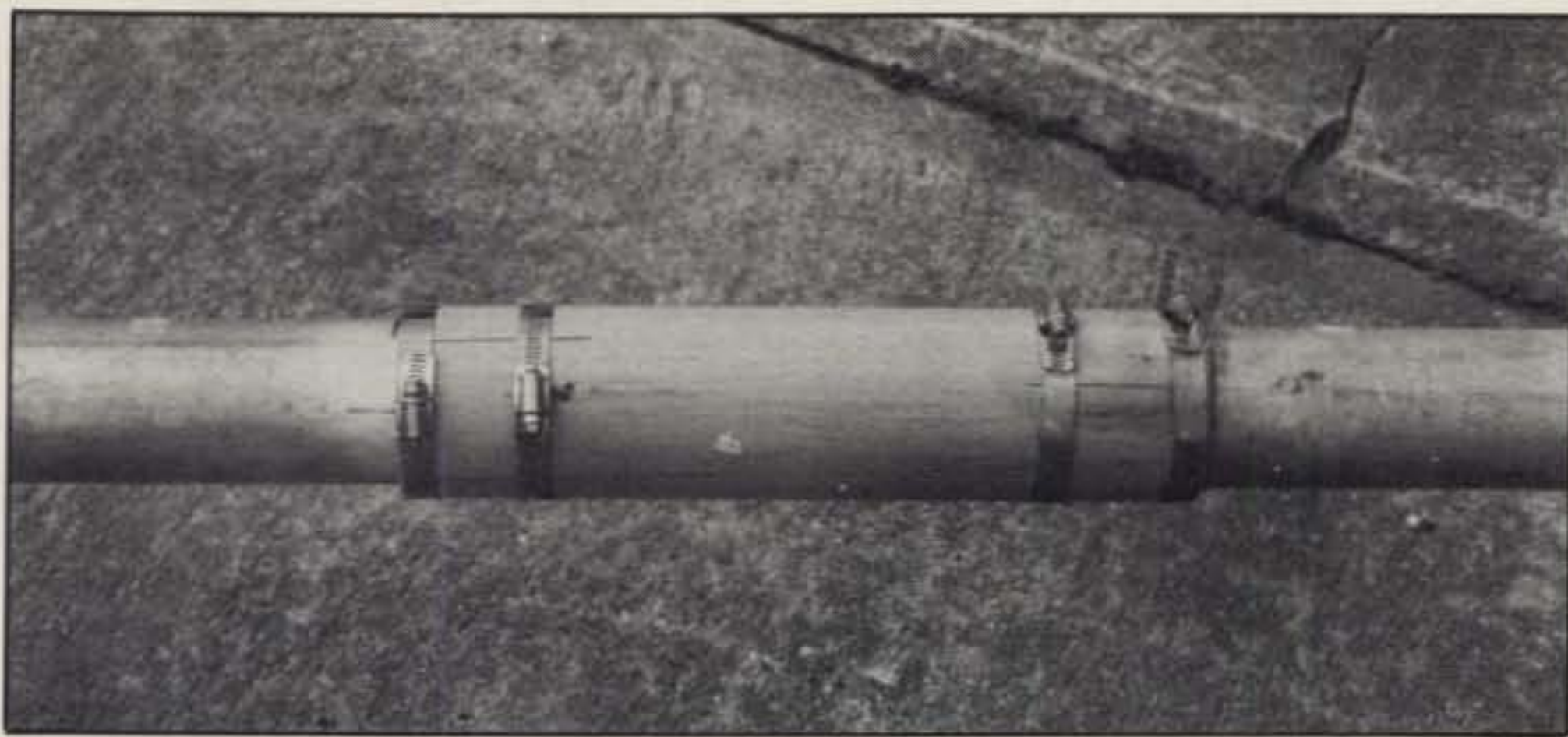
Photo 2— The method of splicing two sections of tubing together.
