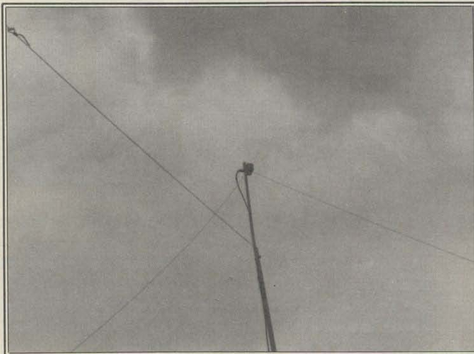
The MDS is a relatively inconspicuous antenna. A plastic enclosure was used at the junction of the antenna legs and the transmission line to weatherproof the junction and as a means of attachment to the mast. The single wire going off to the left is a part of another antenna system, not the MDS.
