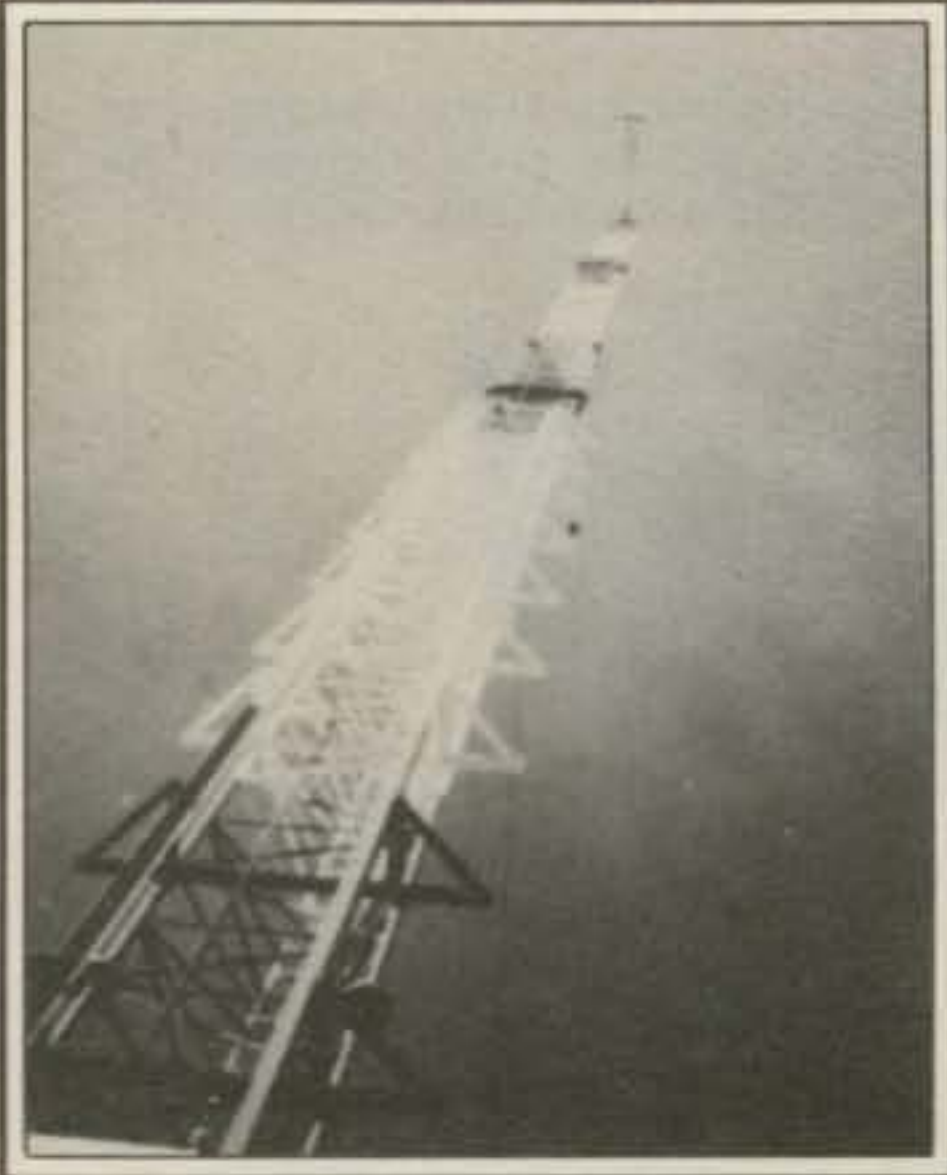
This is one of the 400-foot antenna towers used by WWVB and WWVL. Each antenna is a top loaded vertical supported by four guyed towers arranged in a diamond. The structures are free-floating and completely insulated from the towers. Electrically, the antennas act like high-Q capacitors tuned to the operating frequencies of 20 KHZ (WWVL, now off the air) and 60 KHZ (WWVB). (Photo courtesy NBS)
