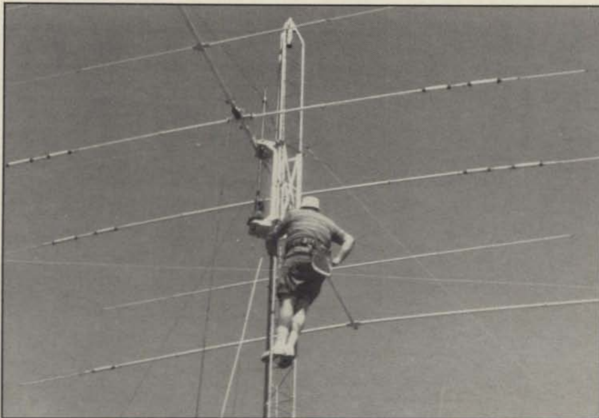
Photo H. The TH7 resting on the Hazer, allowing easy lowering of the antenna to mount it permanently in place.
