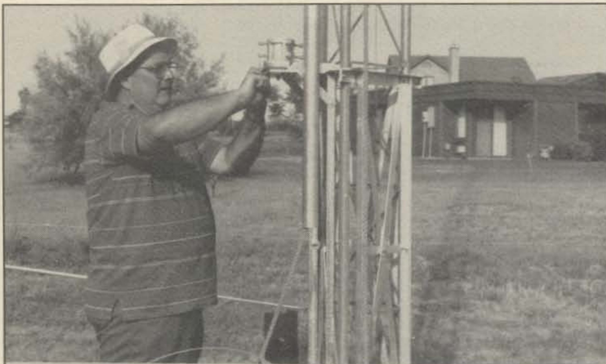
Photo I. N@JW mounting the optional thrust bearing onto the Hazer. The bearing significantly enhances operation of the system.
