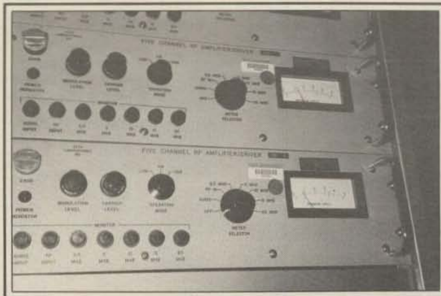
This is a close-up of two of the five channel RF amplifier and driver monitoring units.
