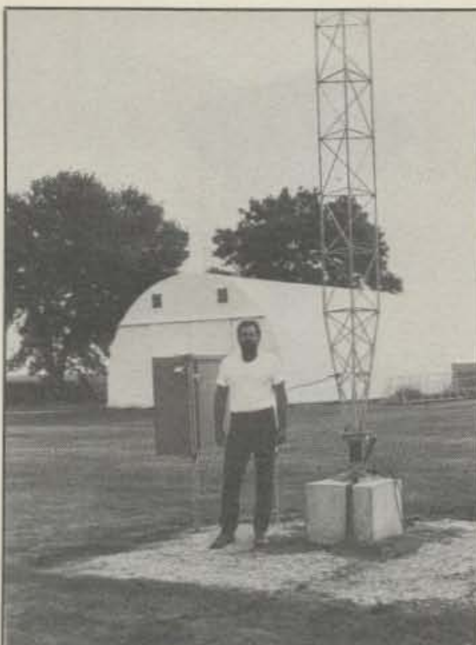
Top USA phone Jerry Rosalio, WB9Z (ex-WB9HAD) at the base of his 160 foot insulated radiator. It has 120 radials using 16K feet of wire. He listens on a high inverted Vee and eight 1000 foot beverages.
