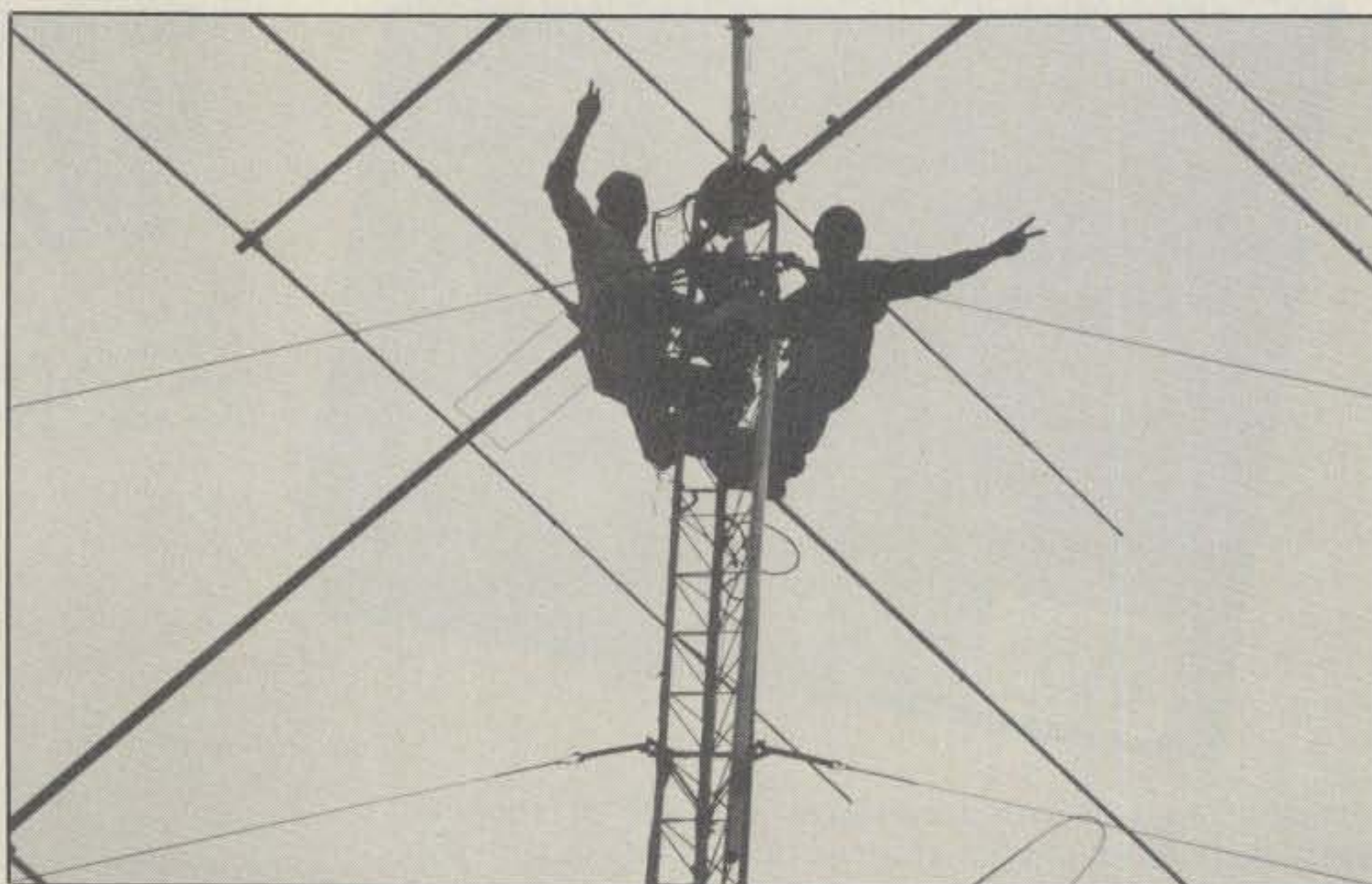
Photo 1—Beginning the disassembly process of the stacked arrays.
