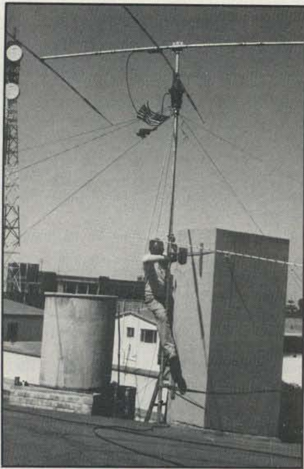
Here's Bill, KC1AG, tightening up the mast for the A-3. All of those guy wires were necessary, as we found out.
