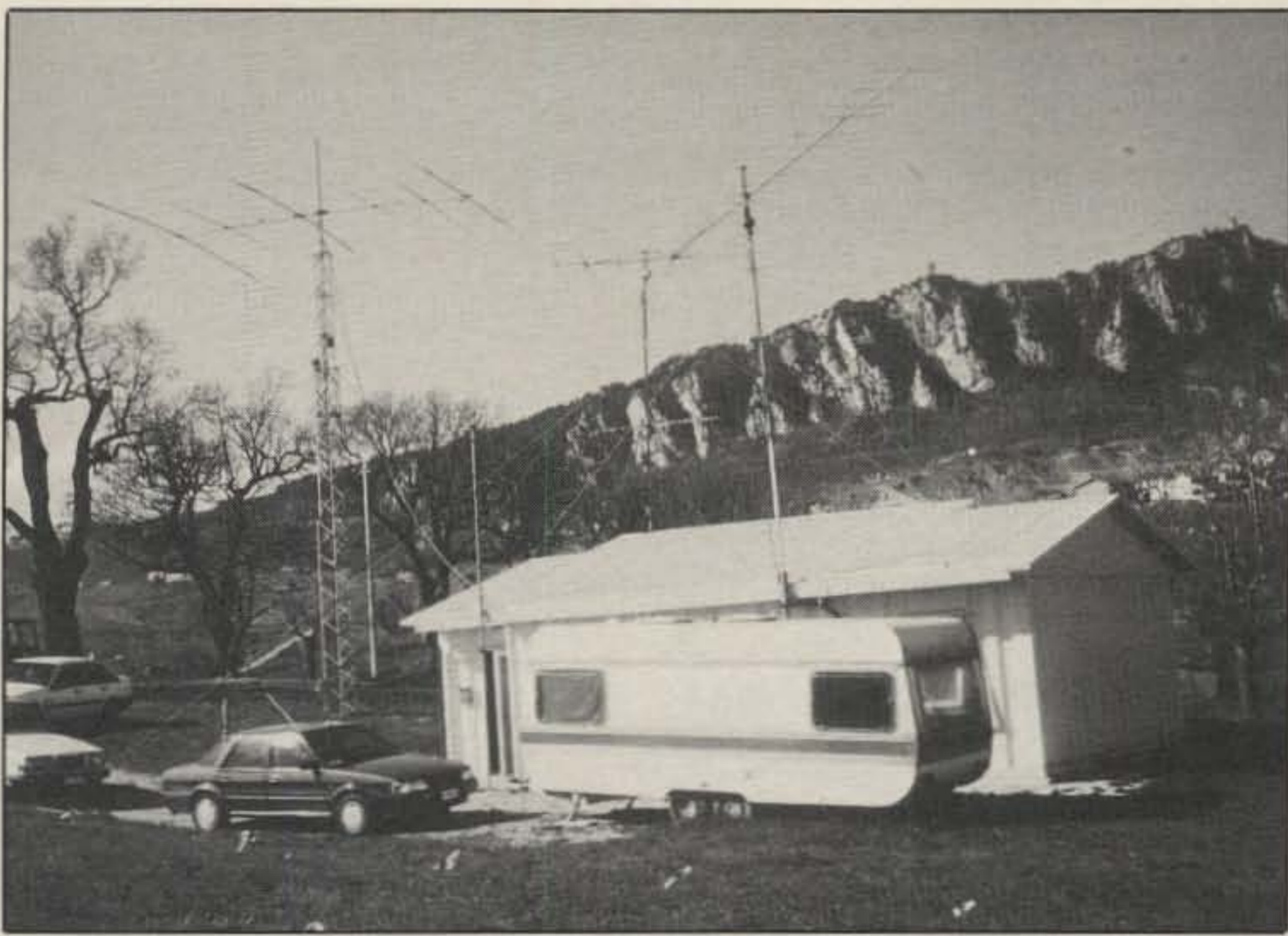
Outside view of ARRSM Headquarters. On the 9 meter tower is the TH6DXX, inverted delta loop for 7 MHz, and the inverted Vee for 3.7 MHz.
