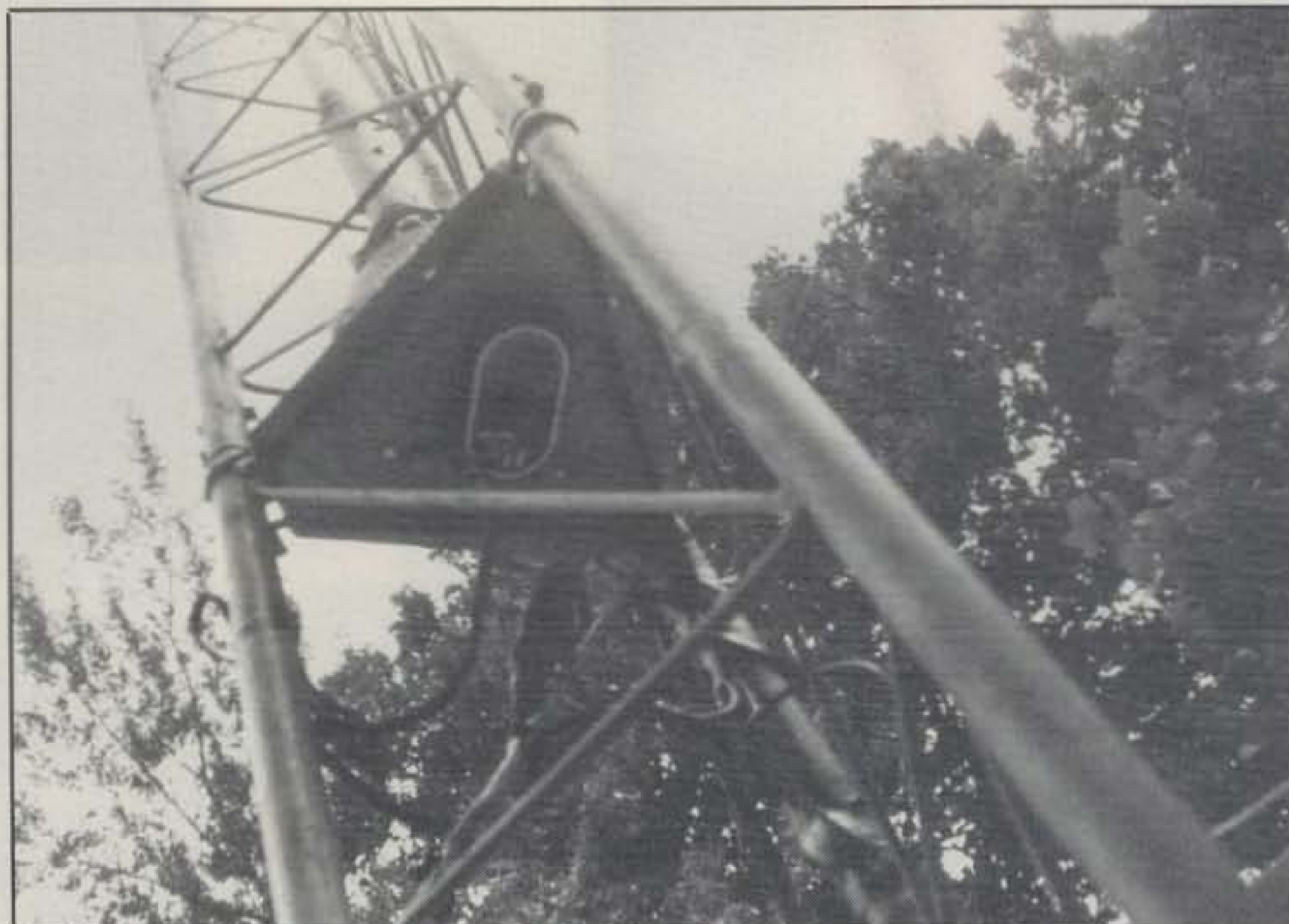
WA0KKC's electric engine-block heater is situated under the rotor and can be turned on as needed from the shack.
