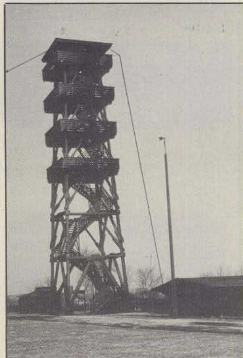
Top West German CW multi-op DK5WL antenna and shack. Other op was DK5WN, and they had a packet connection. They were tenth World-high multi-ops.
