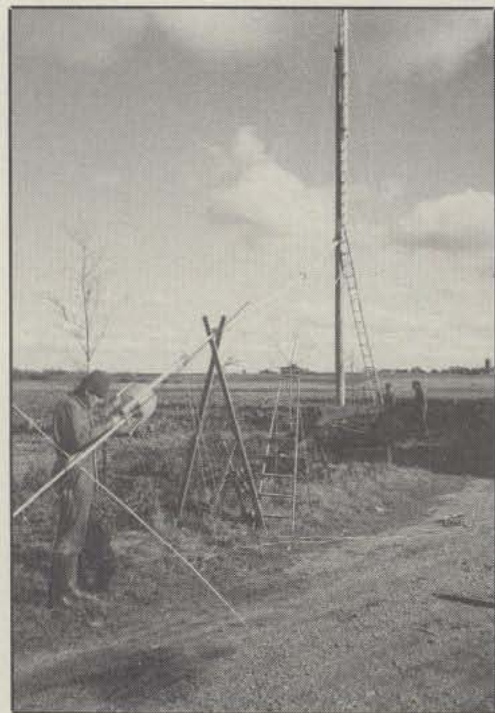
Adjusting top load of OZ1FTE 25 meter high vertical. When operating, there were many radials fanning out from where the top of the tall ladder shows. This station posted the highest Denmark phone score.
