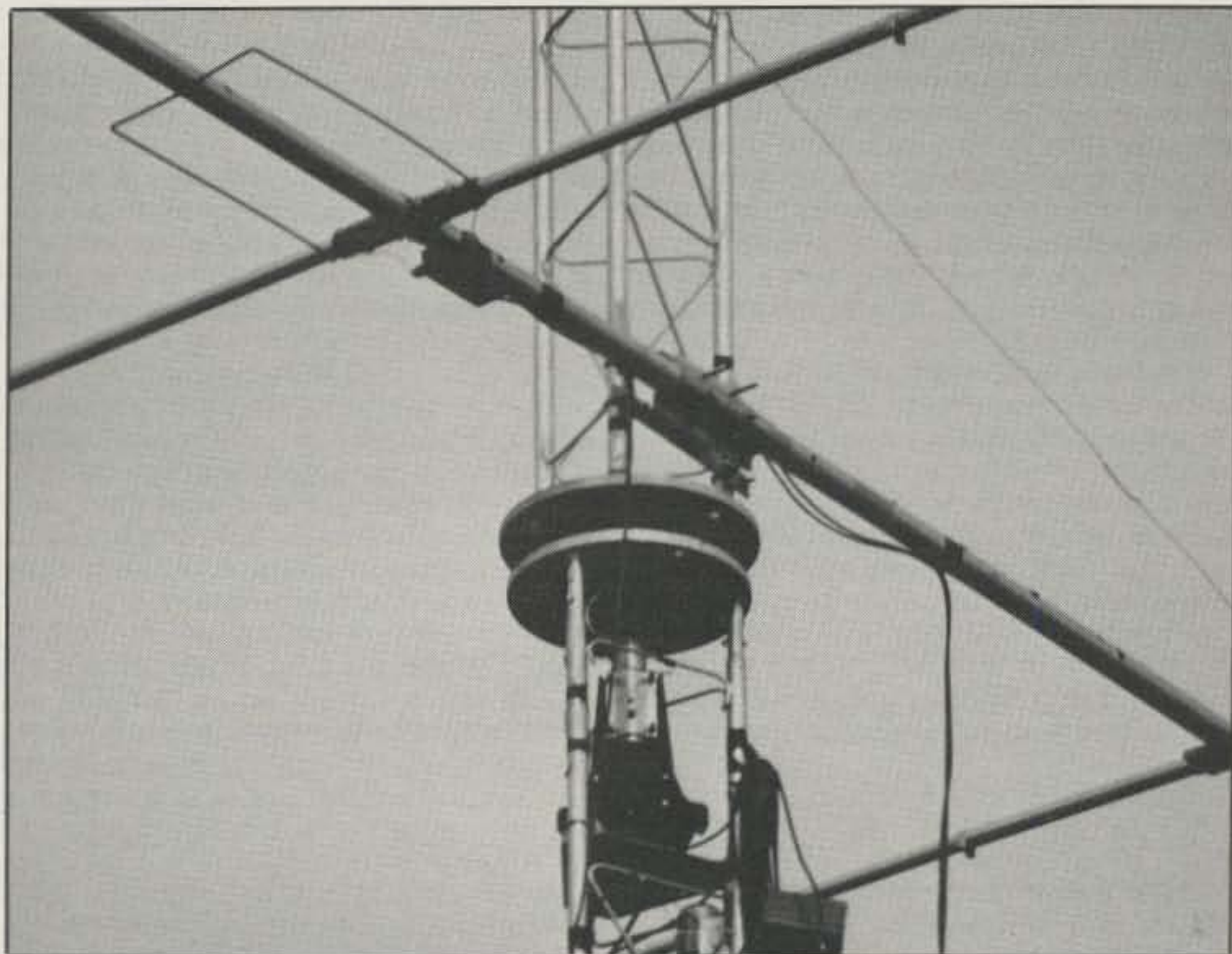
This photo shows the Rohn 25G rotating base assembly at the 60 foot level. The assembly consists of two round steel plates with a large bearing installed between them.
