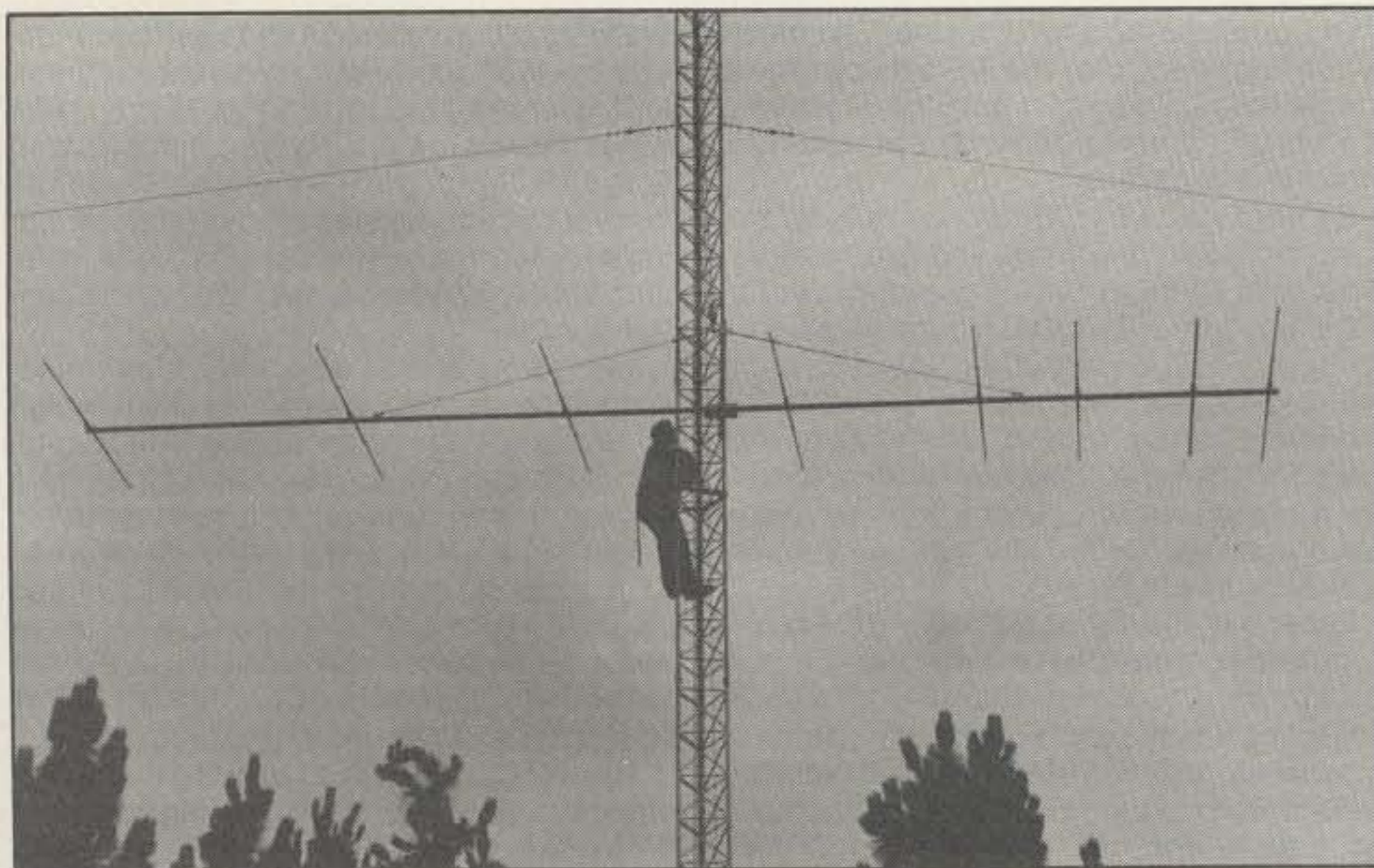
Shown in this photo is DX Engineering's new 6DX-8, an 8-element Yagi on a 2 inch diameter, 36 ft. boom for 6 meters that offers 12 dB free-space gain. We first covered DX Engineering's product line in last July's column; increasing acceptance of the antennas has prompted expansion of the product line to cover both 40 and 6 meters. (Photo via Bill Sattler, N0XX/7)
