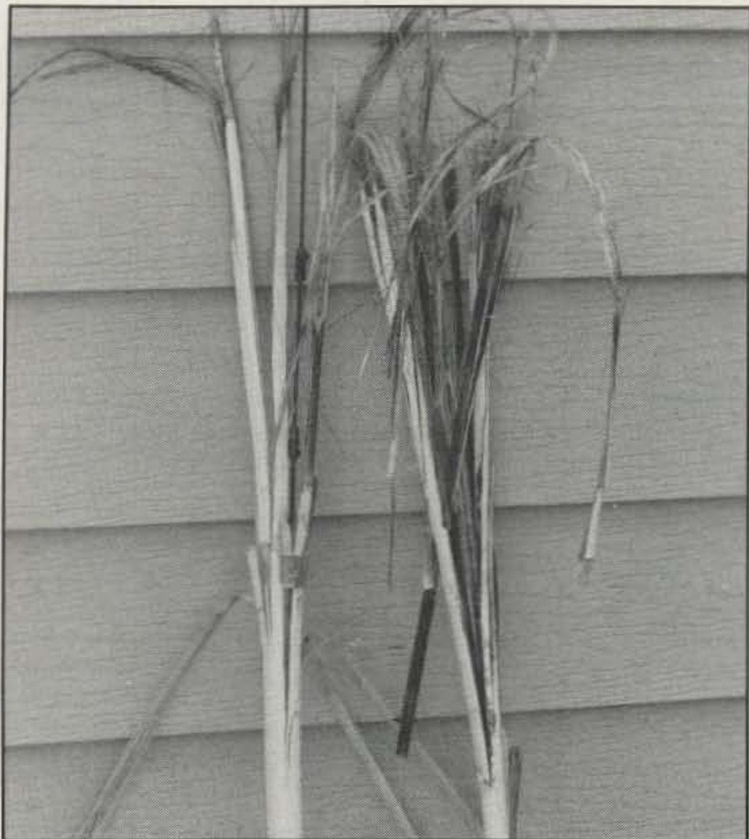
Lightning literally blew the antenna to Hades. The antenna proper, the metal sections, ended up as small balls of metal in parts of the antenna.
