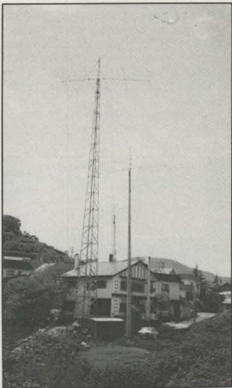
JA8EAT has crammed five large antennas on three towers onto his small lot. The big tower supports a 6-element 40, 20, and 15 meter triband beam at 132 feet, with an 80 meter rotatable dipole above that. Other antennas include a 4-element 20 meter monobander and a 5-element 15 meter monobander at 66 feet, and a 5-element 10 meter monobander also at 66 feet.
