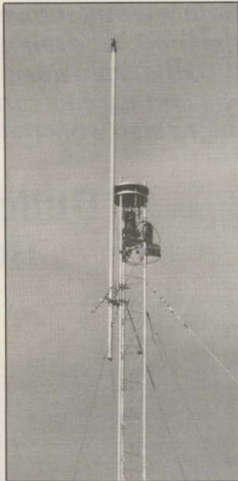
This is what it looks like when the rotating base unit is installed. The switch box can be seen to the right.
