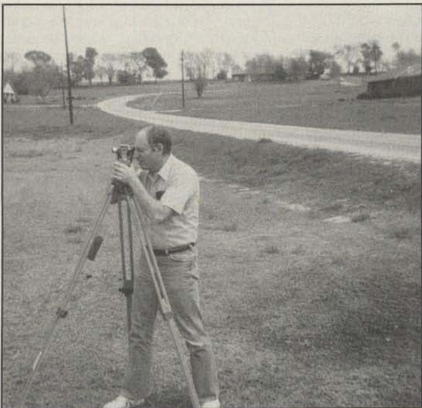
Dick Weber, K5IU, using the theodolite to level the tower during assembly.
