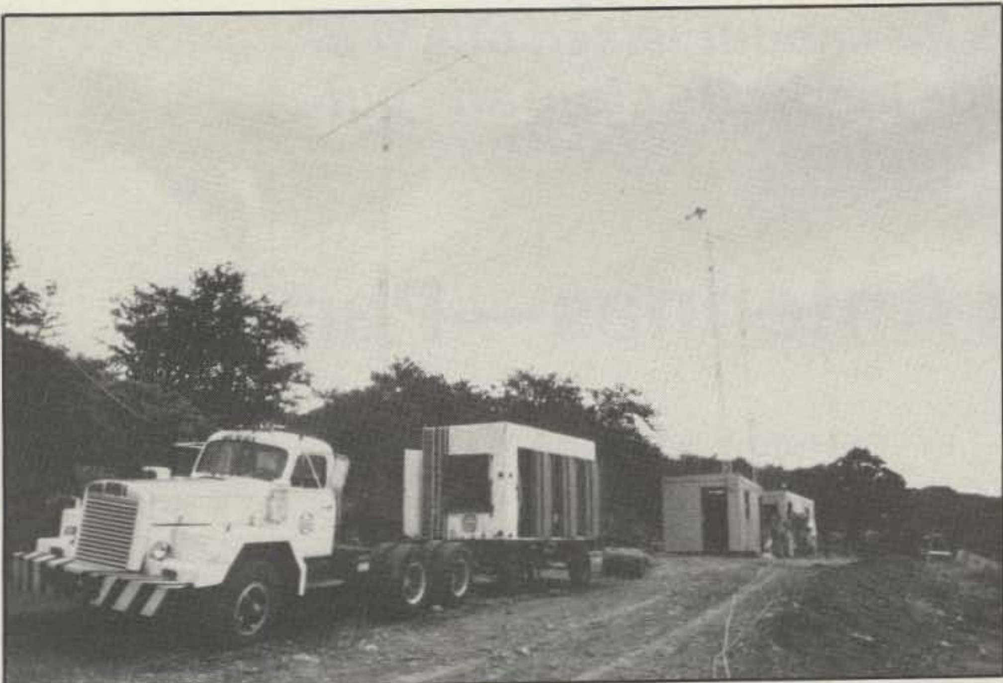
The 300 KW mobile generator being trucked to the operating site.
