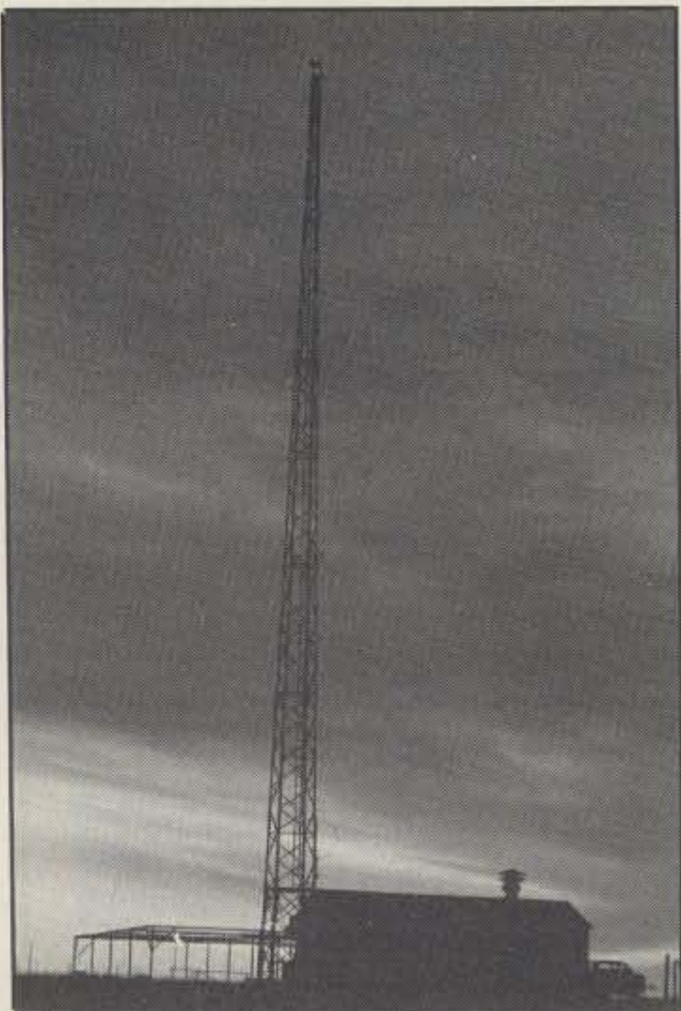
Sunset at WS7W, Wyoming. Shown is the 140 foot insulated tower with 4500 feet of radials 10 feet above ground.
