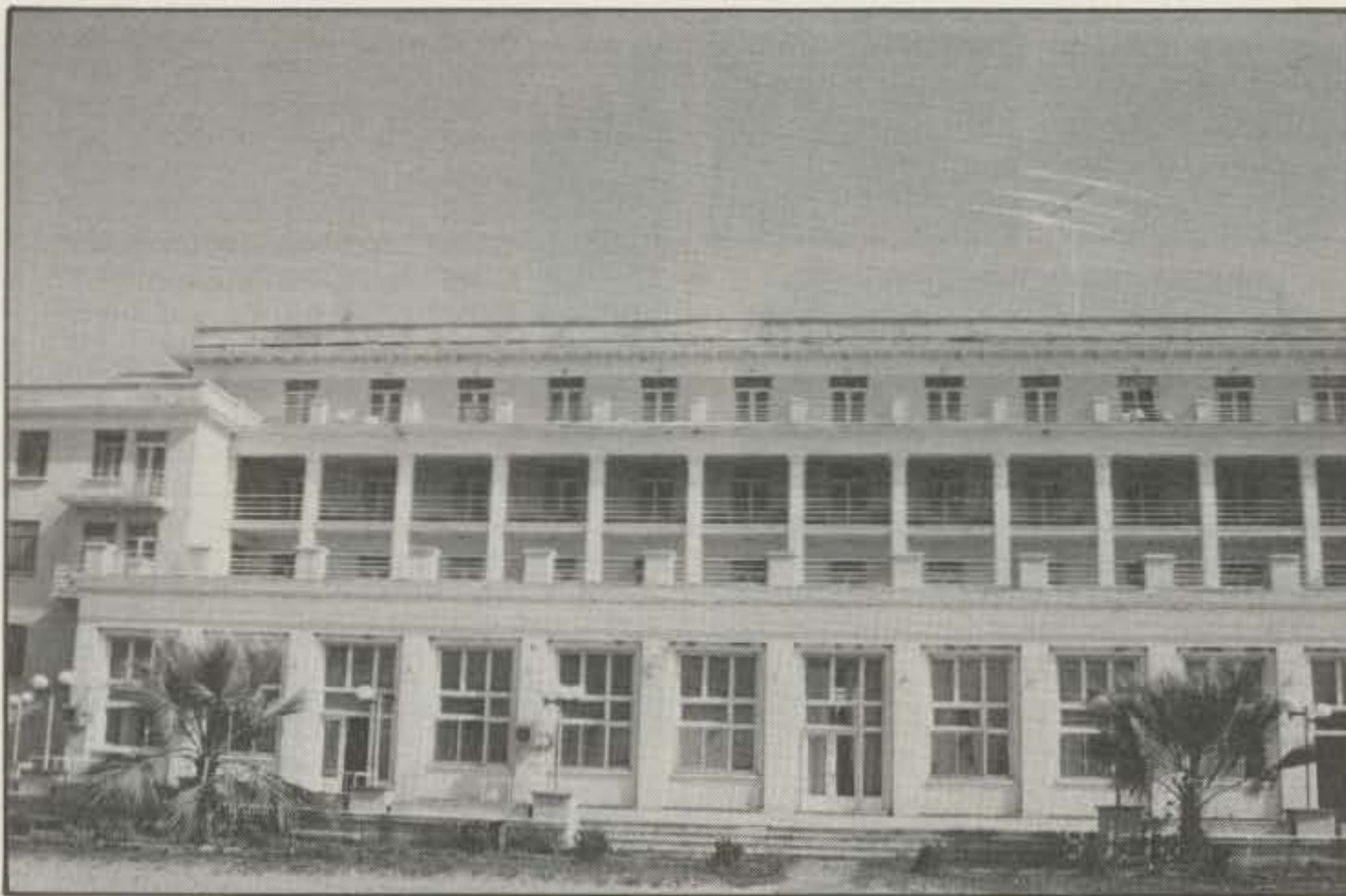
Toward the end of the ZA1A operation another site was established at the Adriatiku Hotel in the seaside town of Durres.
