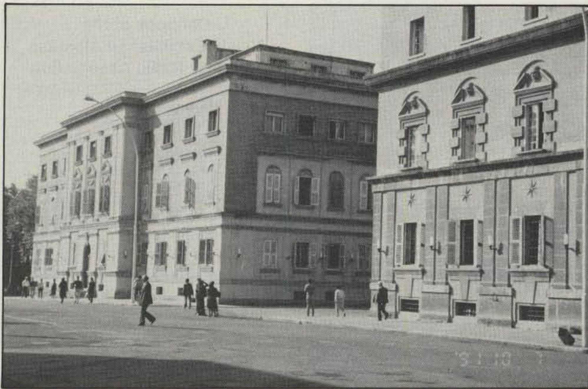
These defense buildings located right at the heart of Tirana provide a solemn framework when the establishment of amateur radio in ZA-land was first discussed.
