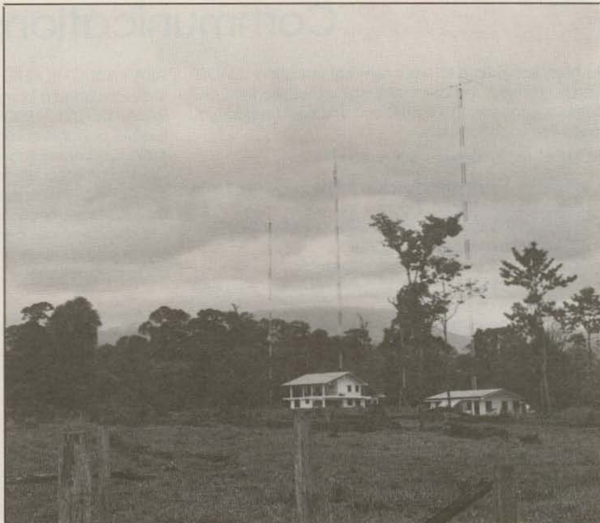
The growing antenna farm at Carlos, TI4CF's QTH.
