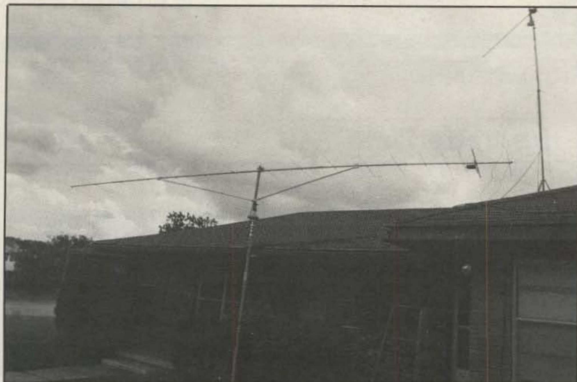
The 17B2 mounted on the push-up TV mast, almost ready to be raised.
