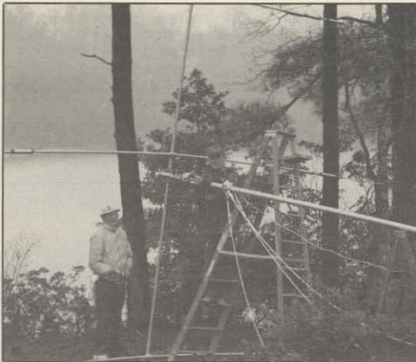
Here the antenna gets some last-minute tweaking from Warren Bowers, WB4MRH, and Harry Kepley, N4THN, before it goes up.
