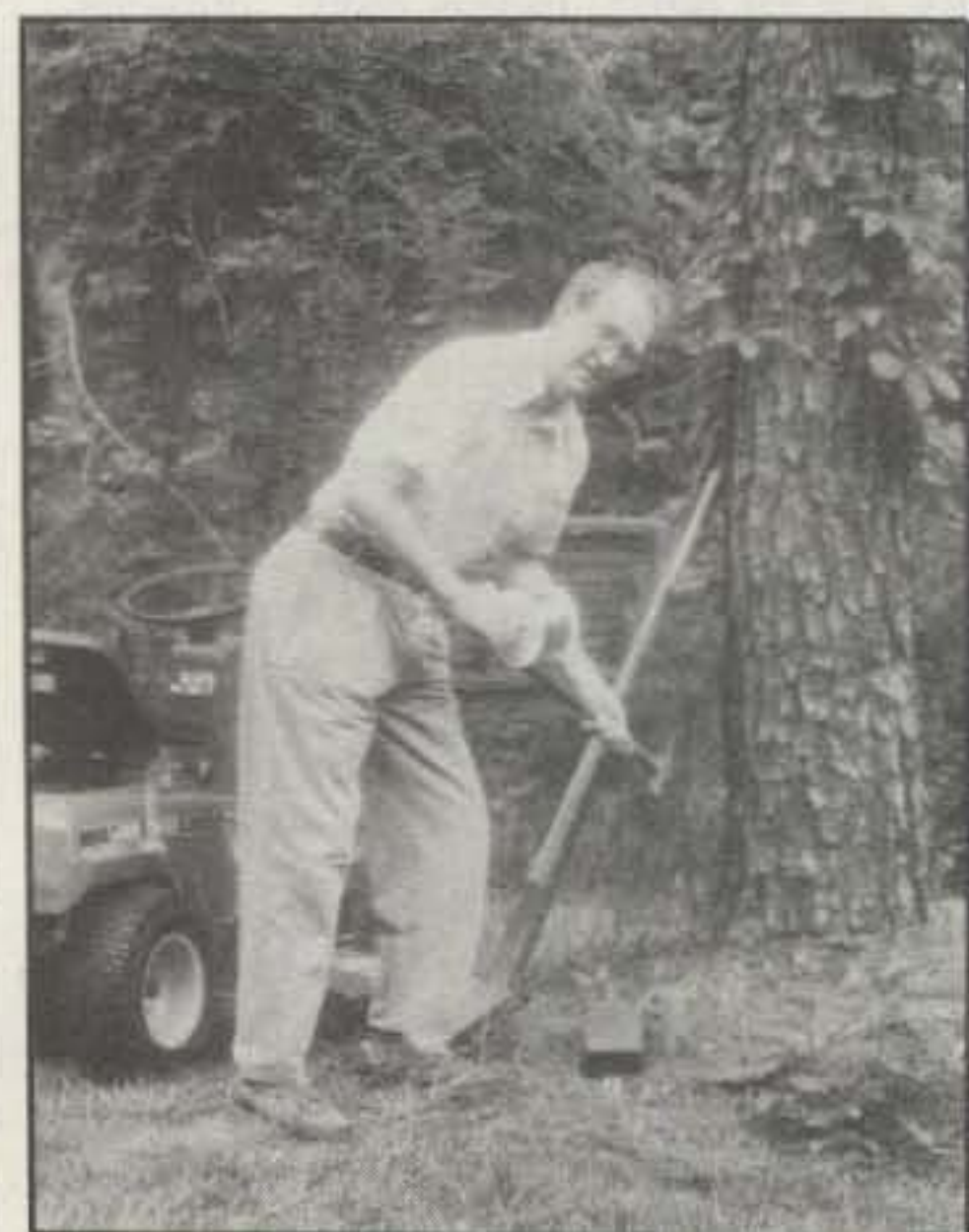
Photo C— ND1W "planting out some radials." The tuning capacitor for the vertical is in the water-tight box, which is normally covered by pine needles.
