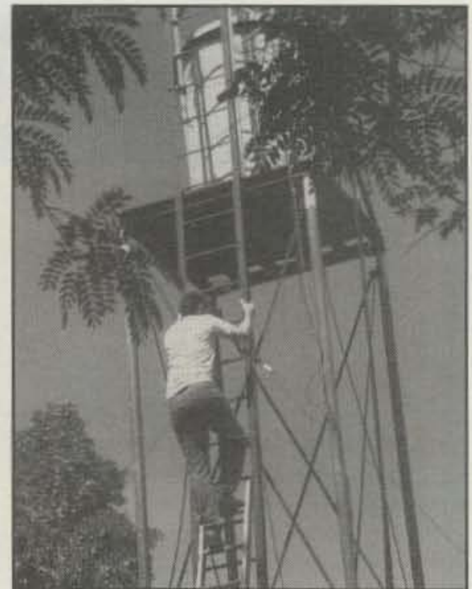
Paul Young, K1XM, operated from the More Wanted country of the Seychelles as S79S in CQWW CW last year. Here he installs a low-band sloper on an handy water-tank tower.
