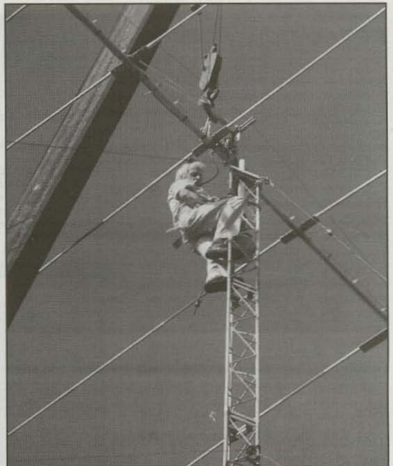
VK9NS ready to connect the big log periodic to the rotor mast. I assume that he is using a very husky rotor, because the wind loading would be, and is, high for this type of antenna.
