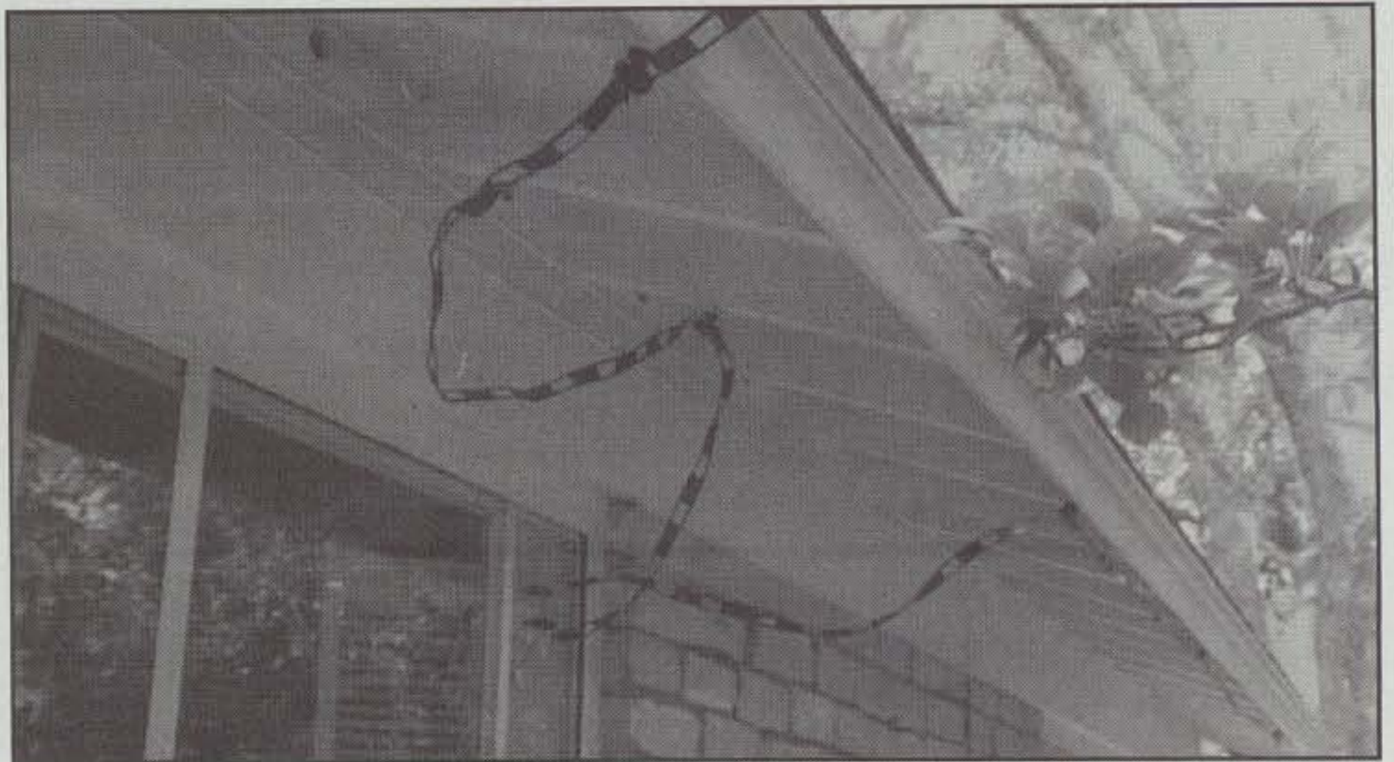
Electric fence stand-off insulators hold these two runs of 450 ohm ladder line in place under the eaves of the house. Note one at right is twisted about twice each 3 feet. The run at left has been replaced with homemade open-wire line.
