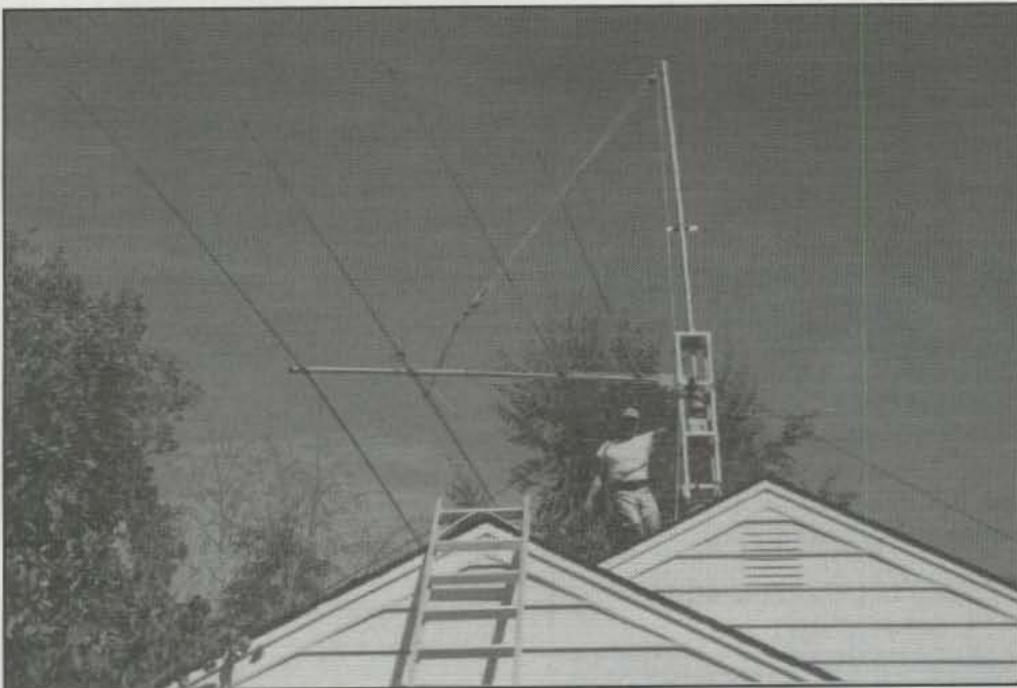
The antenna goes up in two sections. Shown here is the rear half, which contains the reflectors and part of the log-periodic setup.
