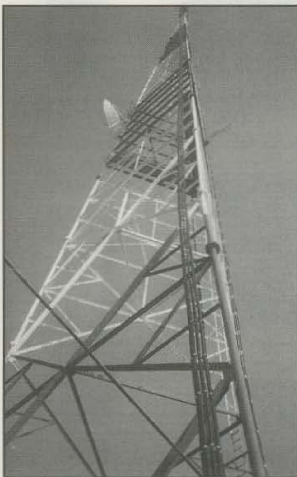
Somewhere up there about 300 ft. at the left of the tower is the G-7 antenna for K4ICT-7.
