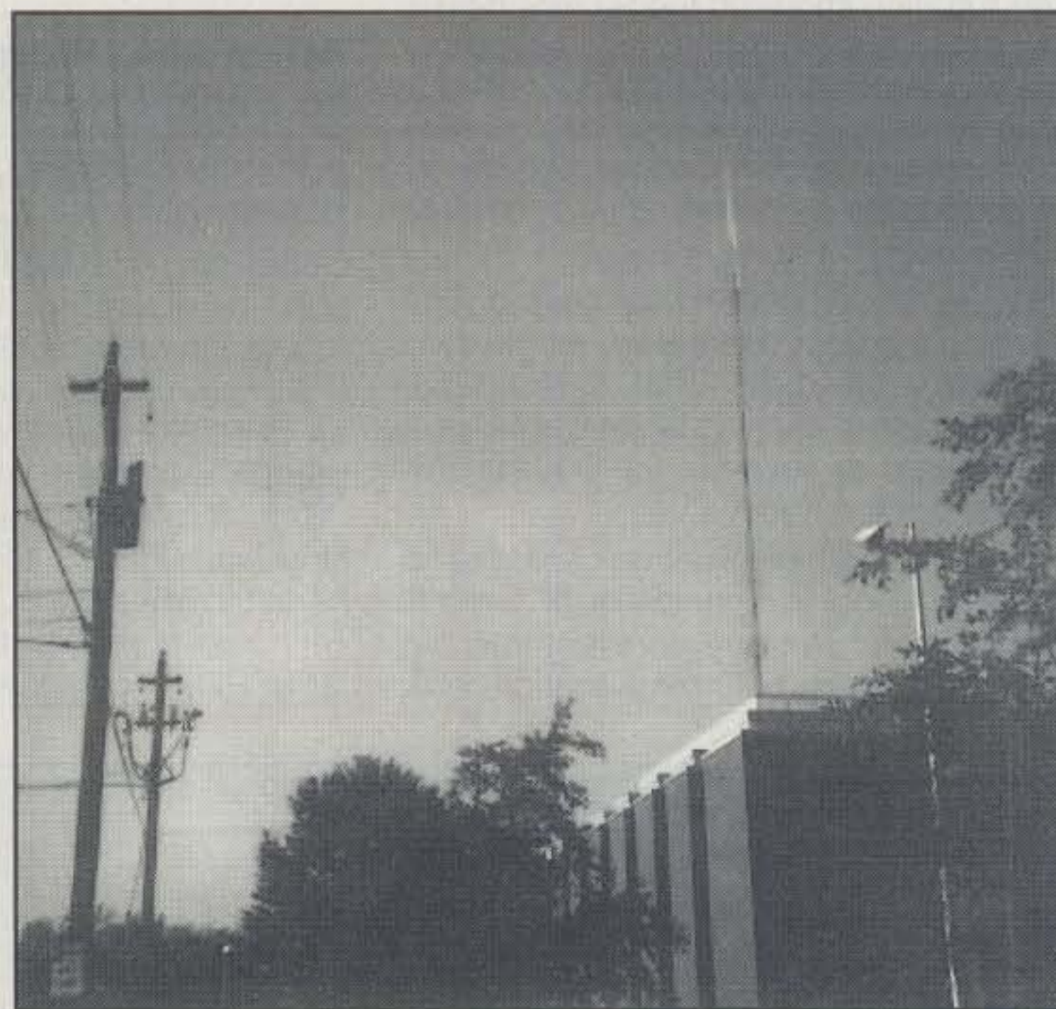
The antenna for SEDAN node "WNC" is atop the hospital at Wadesboro, North Carolina. A well-planned site by the Wadesboro, North Carolina amateur radio group.
