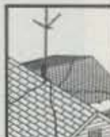
KD4JKX-8/ILM antenna near Wilmington and Carolina Beach, North Carolina. The quads look inland to handle traffic into the Southeastern Emergency Digital Association Network's system. When hurricane season begins to threaten the coast, these nodes will become super active.
