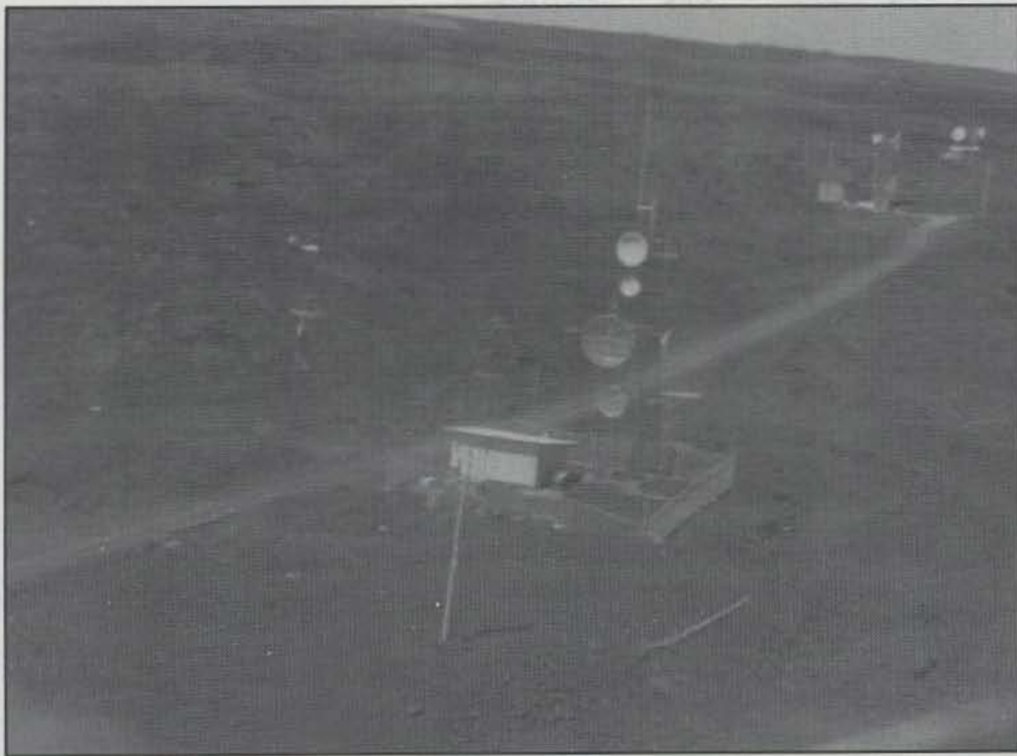
Aerial view of the KH6HME beacon site on the side of Mauna Loa volcano. Paul operated from this site during the record-breaking Hawaii to California opening in July. (Photo courtesy WB6NOA)
