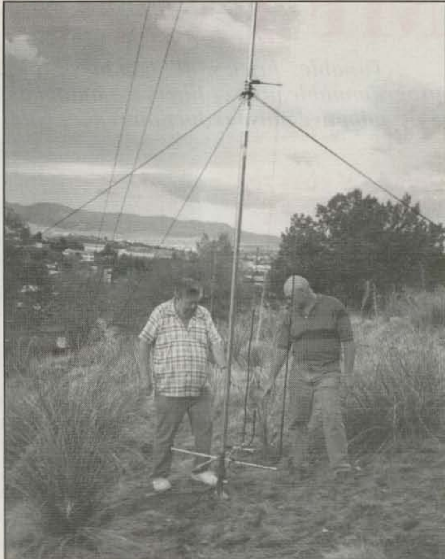
Here are W1ICP on the left and N5NUG on the right. We are checking the final adjustments. An MFJ-249 was used here to get the tuning where we wanted it.
