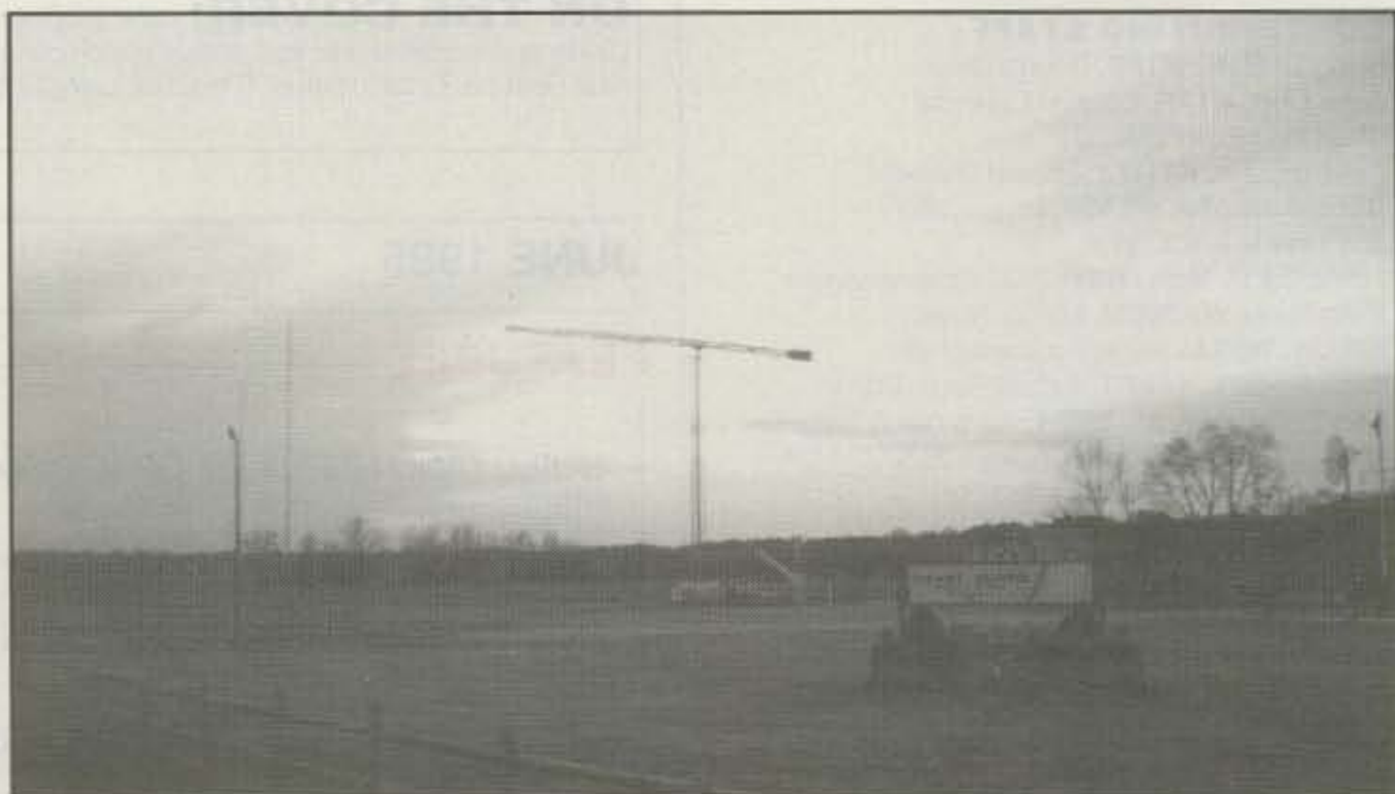
As you approach the U.S. Coast Guard facility; NMN, in Chesapeake, Virginia, the first thing you notice is the large log-periodic antenna in front.
