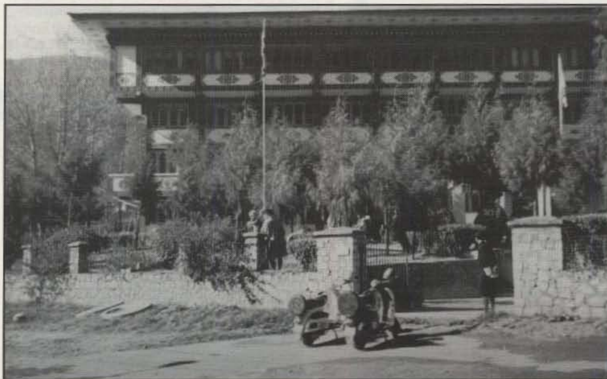
The Ministry of Communications building in Thimphu with the R5 vertical in place.
