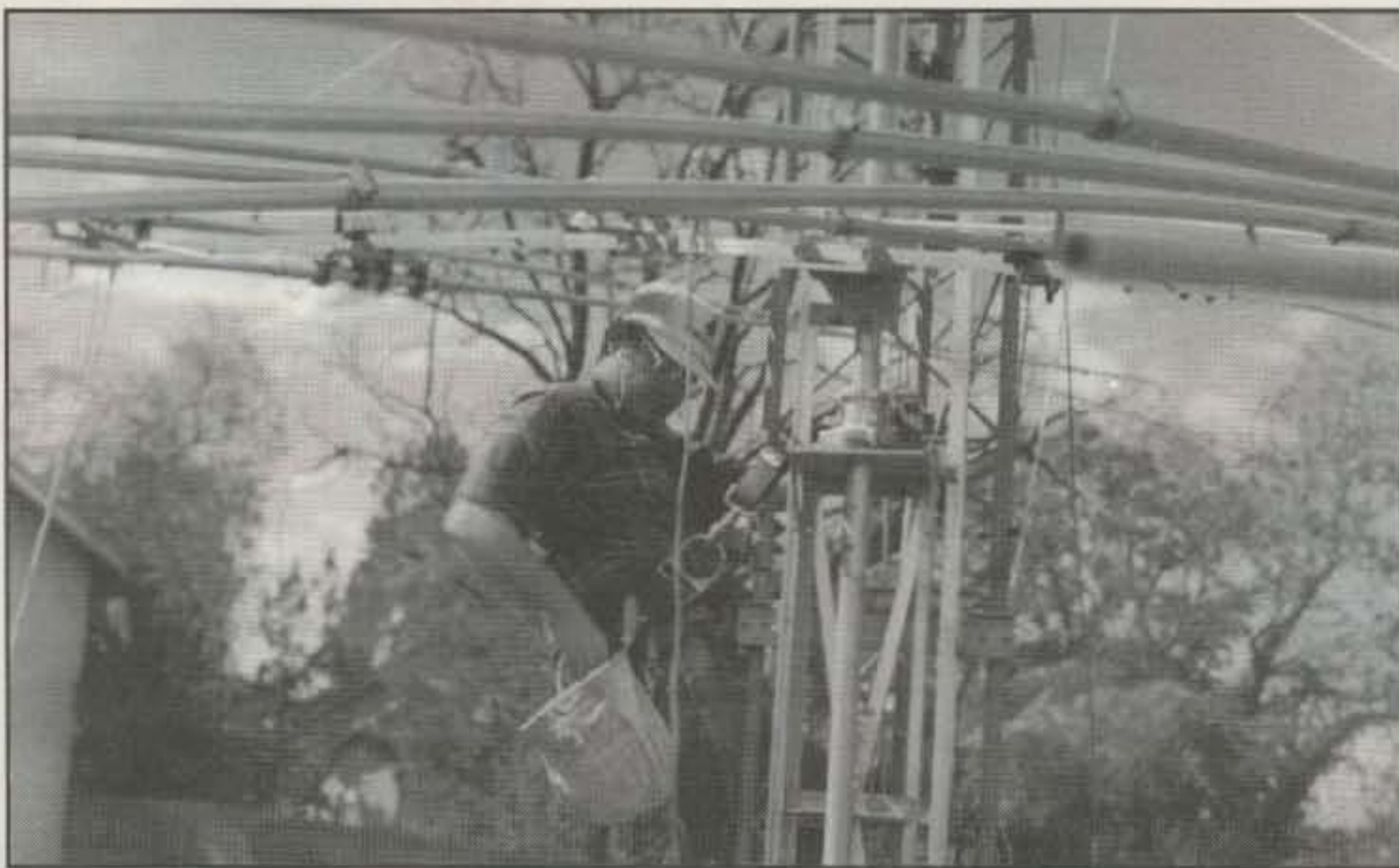
This view shows the top of the carriage and the thrust bearing of the beam mast.
