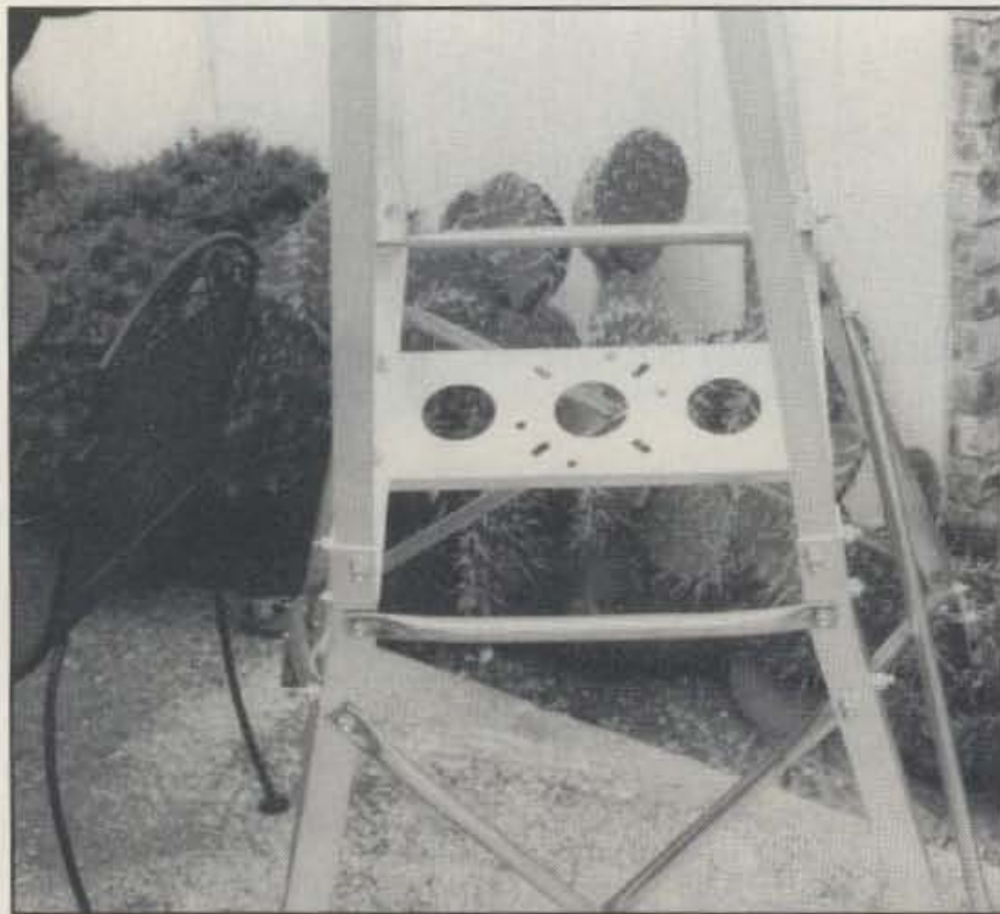
The antenna rotator mounting plate can be adapted for several models of rotator.
