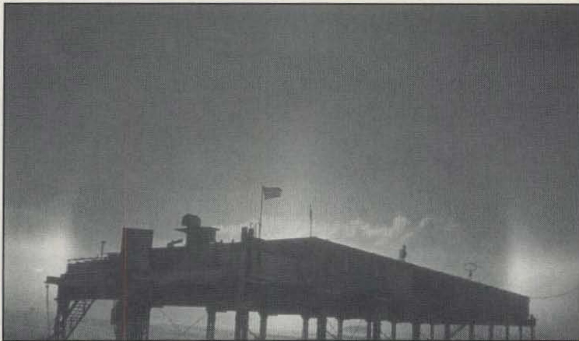
This is a photo of the Accommodation Building at Halley Base, Antarctica. The legs of the building need to constantly be jacked up to keep the building above the rising snow level. The amateur radio station is located in a smaller but similar building known as the Space Science Building, or SSB—an apt place to be. In this view you can see the sun's rays forming a mystical effect around the building.
