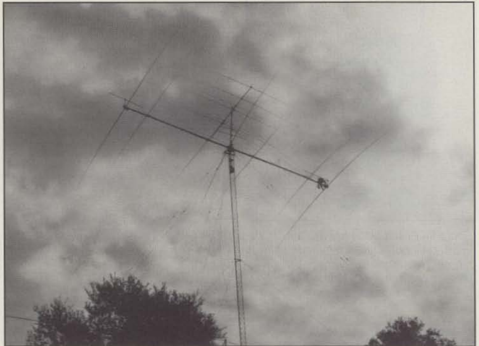
Photo A— Shown here is Paul's 120 foot tower sporting a 3-element 80 meter Yagi interlaced with a 4-element 40 meter Yagi. Atop that is a C3 Force 12 multiband Yagi for the higher bands. If you look closely, you can see Paul on the left astride the tip of the boom adjusting a guy wire.
