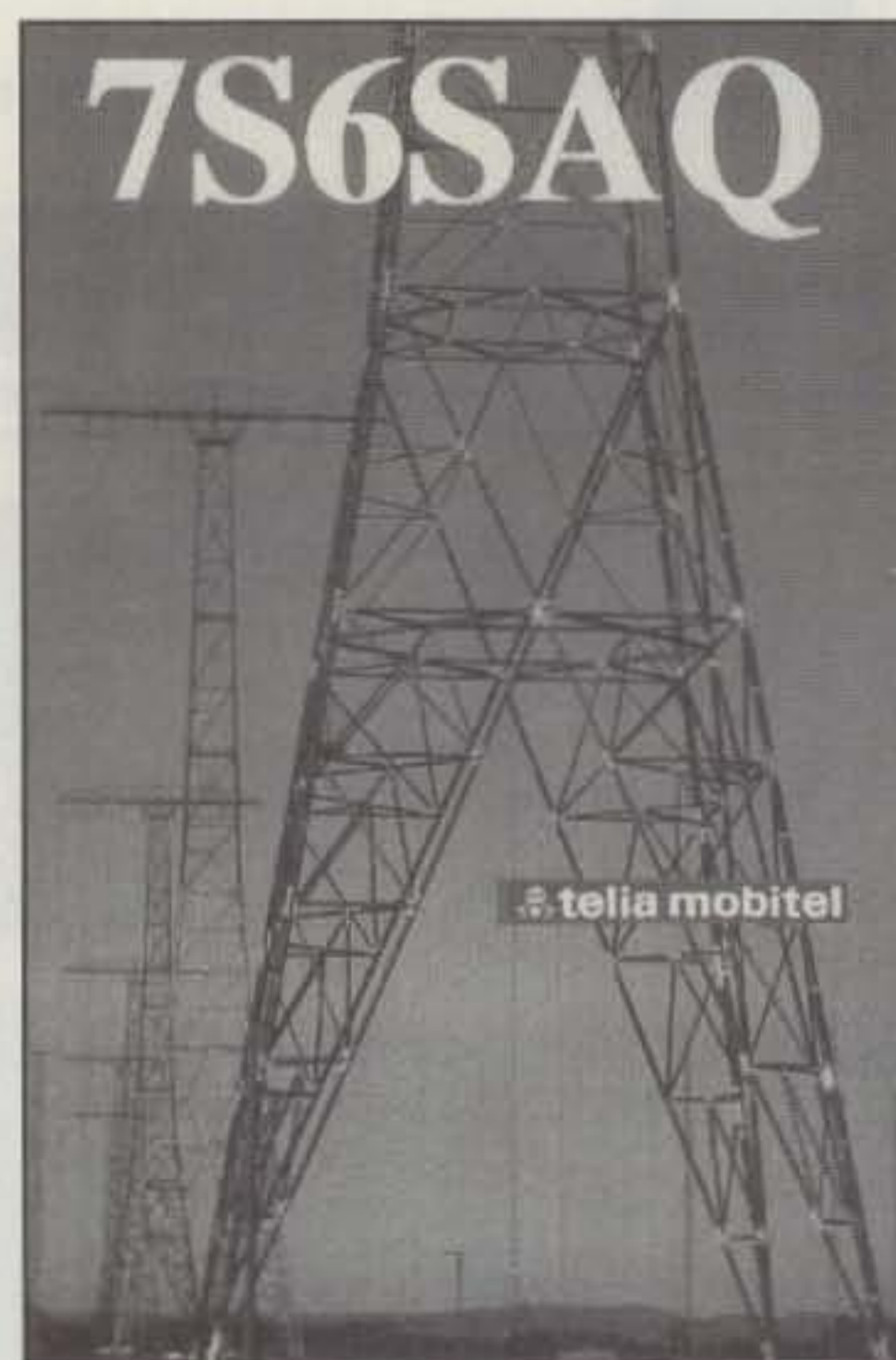
The 7S6SAQ Grimeton station QSL card. The Grimeton radio station, described in the text, is situated on Sweden's west coast. In the mid-1920s it started regular radio transmissions to Long Island, New York, on a frequency of 16.7 kHz using the callsign SAQ. Today the station operates on ceremonial occasions, typically once a year, on 17.2 kHz, using the callsign 7S6SAQ. The site, complete with six antenna towers and a 200 KW transmitter, is managed by Telia Mobitel (Telia AB), a Swedish mobile telephone company, and the radio museum of the Radio Historical Society of West Sweden. (QSL card courtesy Telia AB, Sweden)
