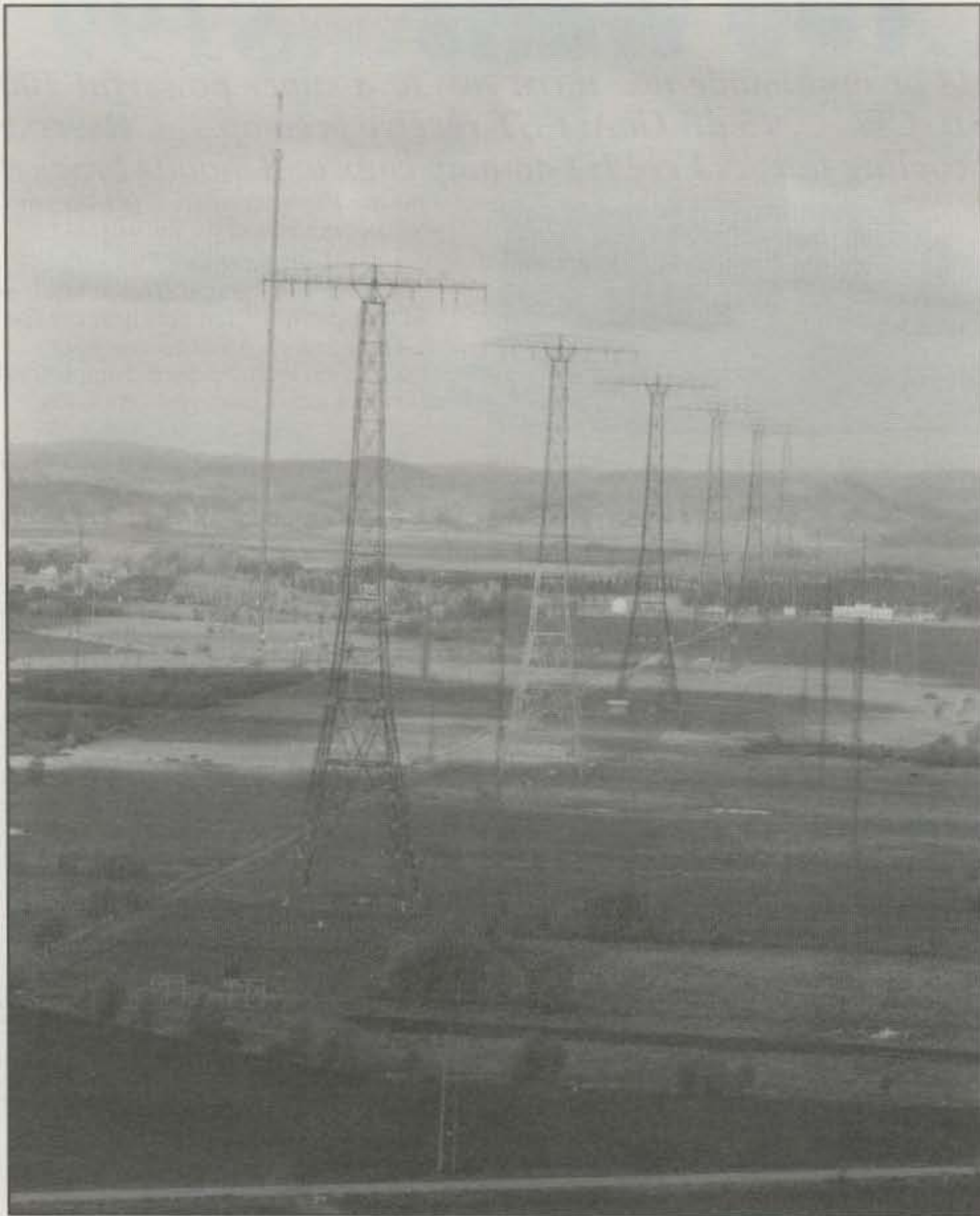
The massive towers associated with the Grimeton, Sweden Alexanderson alternator still are usable. The antenna system has six 127 meter high towers spaced 380 meters. On the top of each tower is a 50 meter long T-arm to carry the 12 wires feeding the six vertical antennas. (Photo courtesy Telia AB, Sweden)
