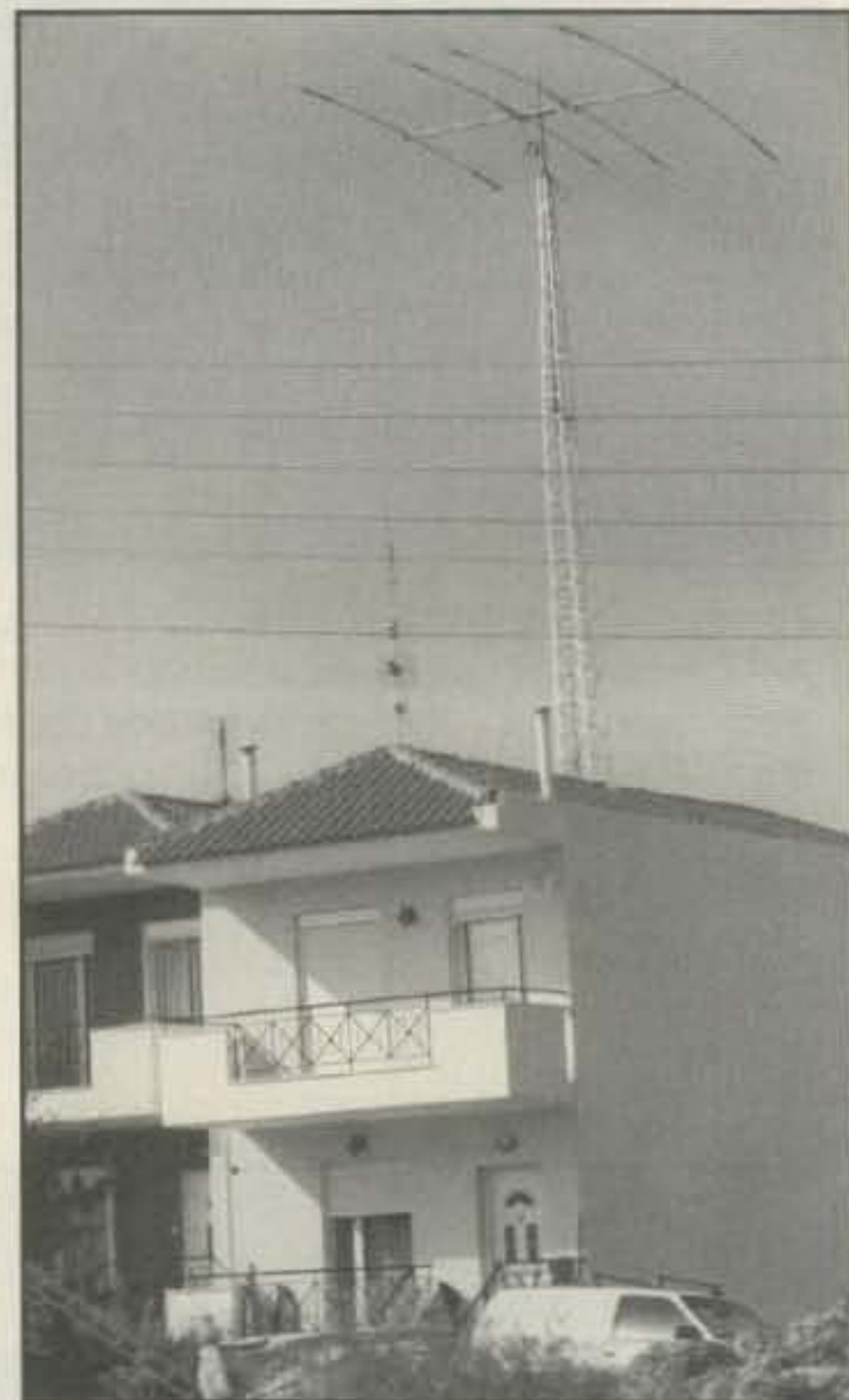
How to put up a tower without much space? Chris, SV2CWY, solved that problem with a homemade tower extending through the roof of his house.
