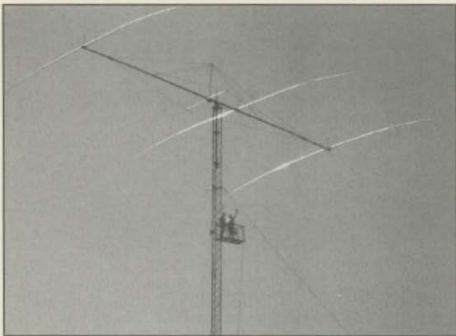
↑ You can judge the size of the array by the two men on the catwalk. The catwalk folds up against the tower when not in use.
