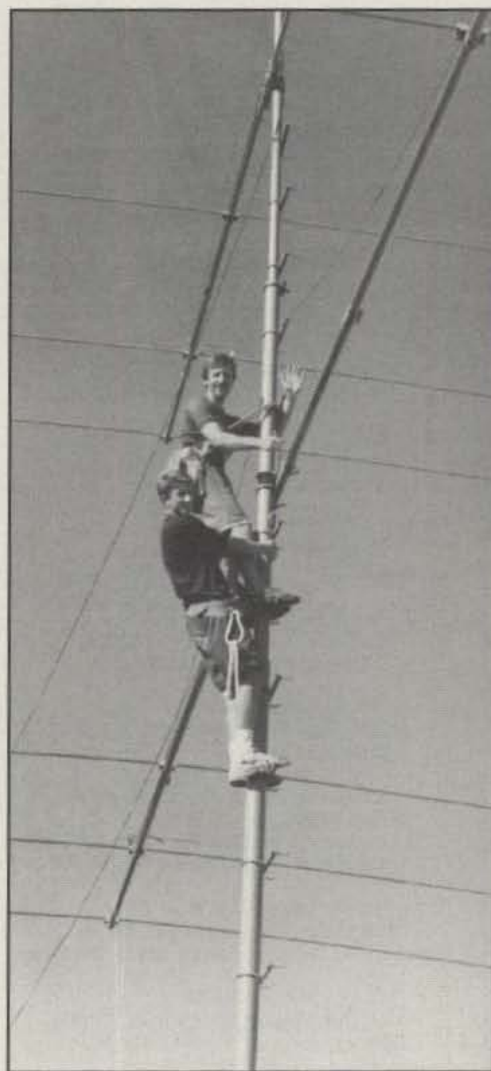
Wes, SP4EEZ (SP4Z), up the tower with his brother placing the homebrew 6-element Yagi on the mast.
