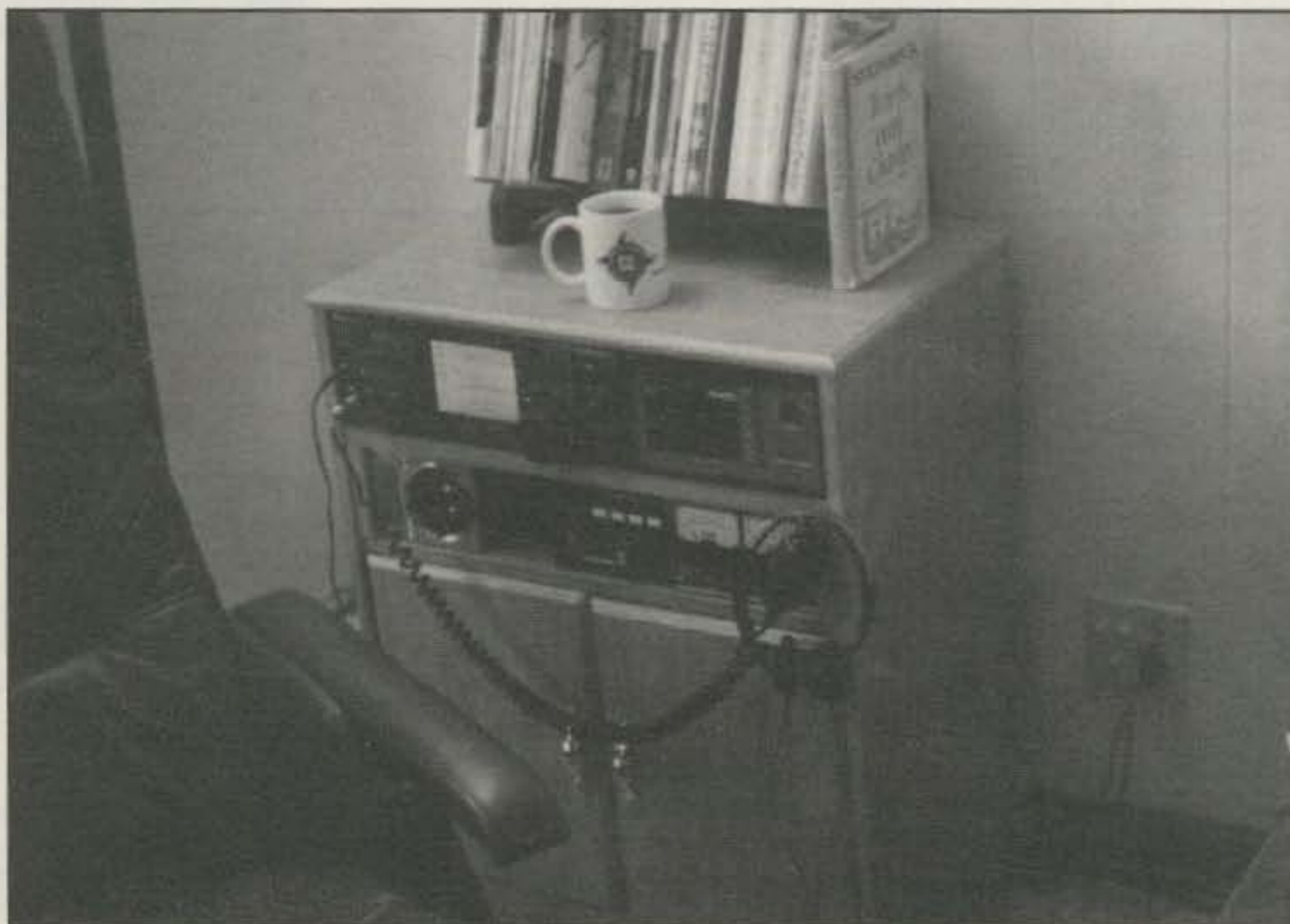
Nary a cable in sight. A cabinet designed for home entertainment equipment was pressed into service for amateur radio. After all, home entertainment can mean a lot of different things.
