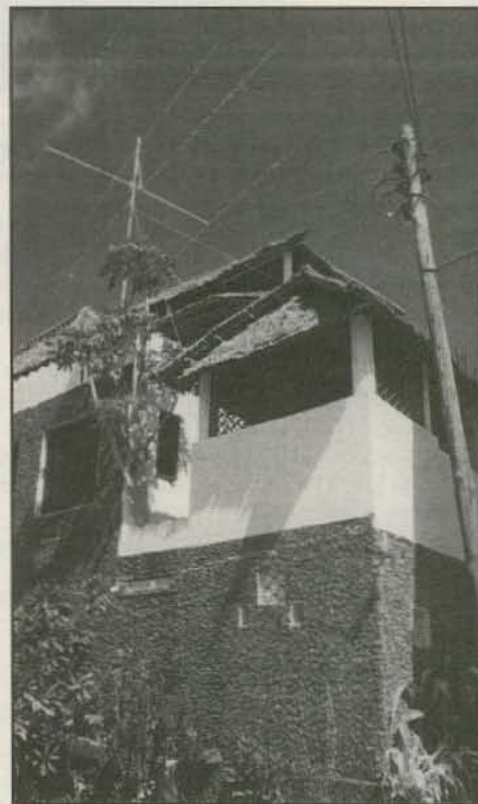
The antennas and the power lines.
